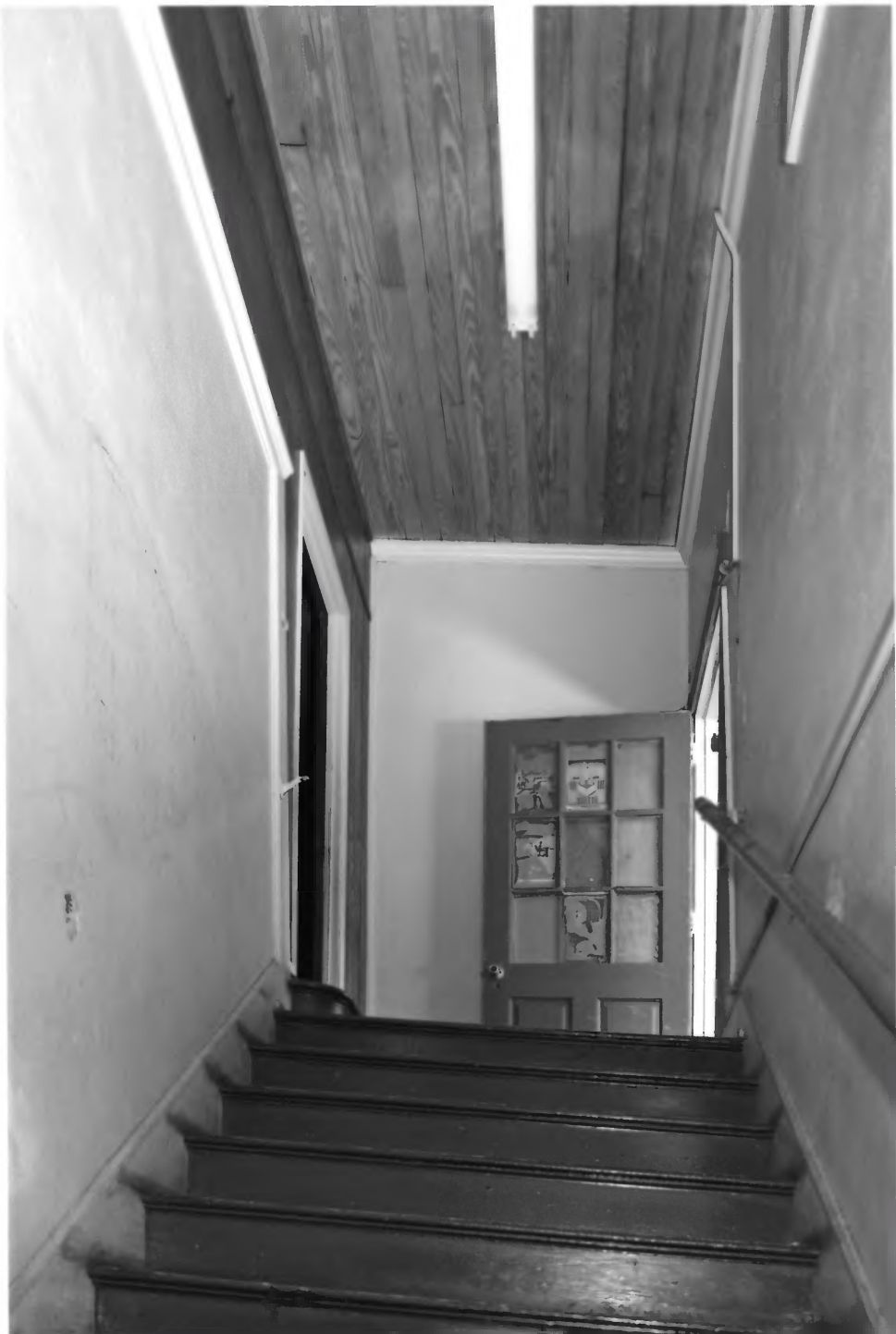
Bacon County School Bacon County, Georgia Photograph 20 of 26
