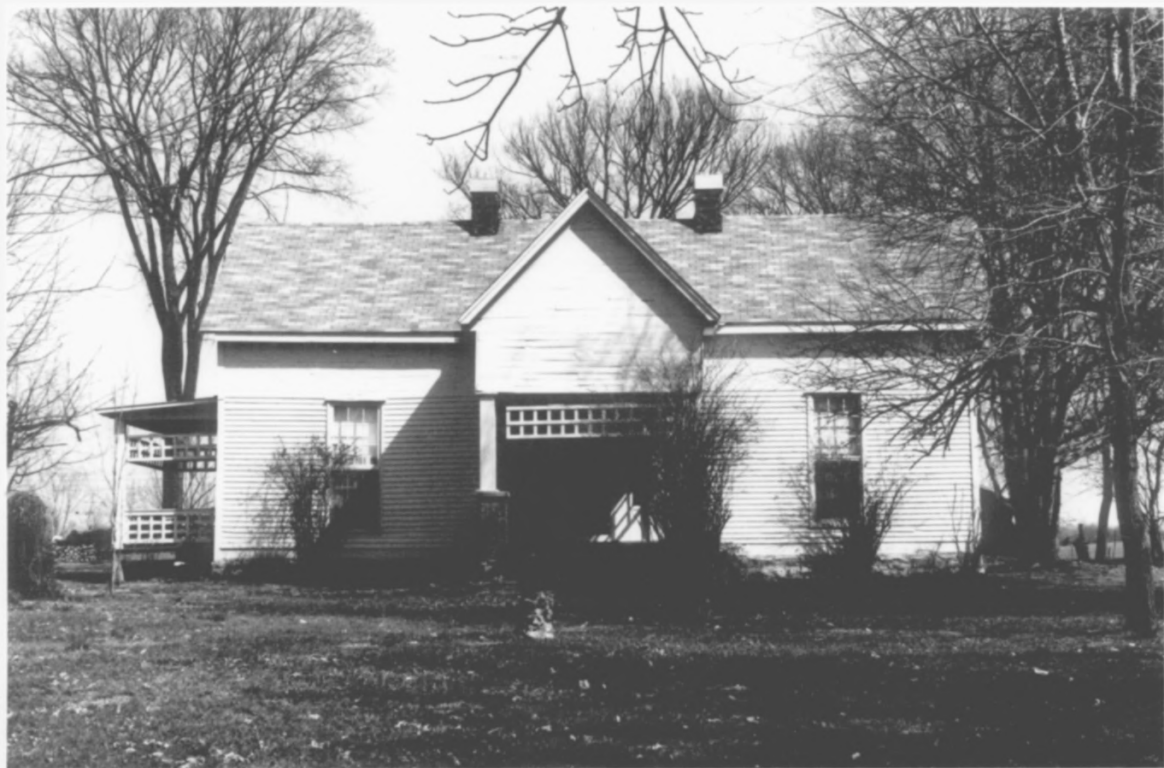
Heidt Tavern / Singleton Residence Wartrace vicinity, Bedford Co., TN
