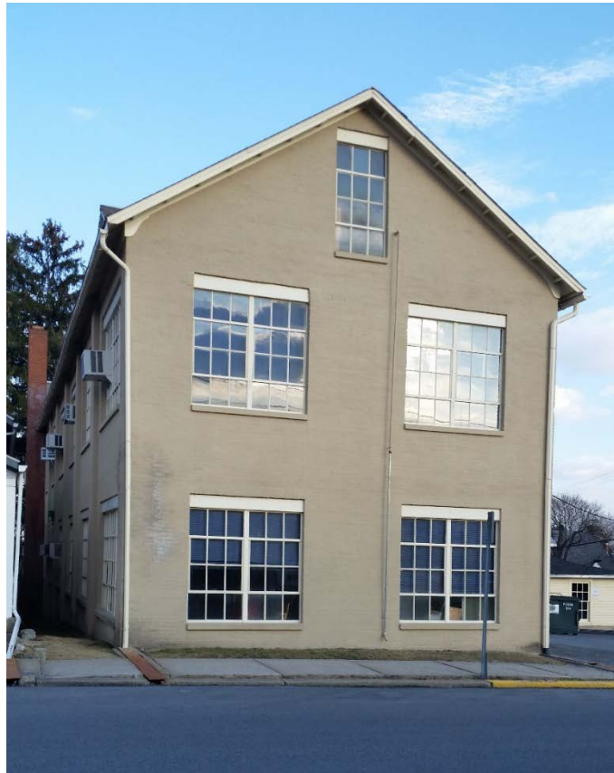
33. Side and back of Manufacturing Building 3. Camera facing east.
