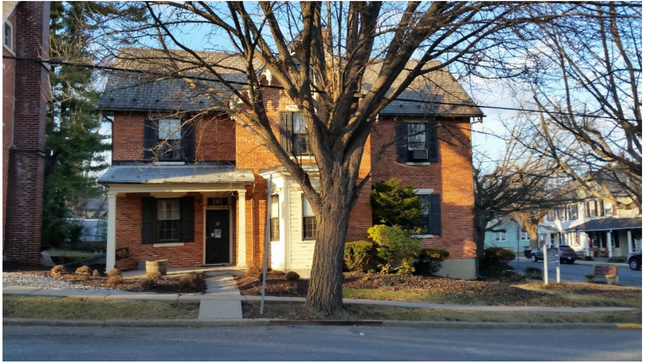
22. Side entrance to the Martin House. Camera facing north.
