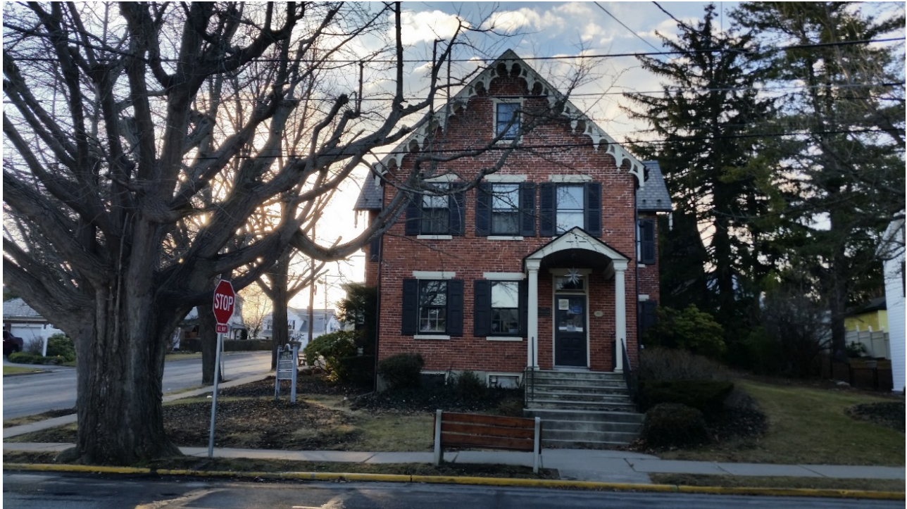
20. Front entrance to the Martin House. Camera facing west.
