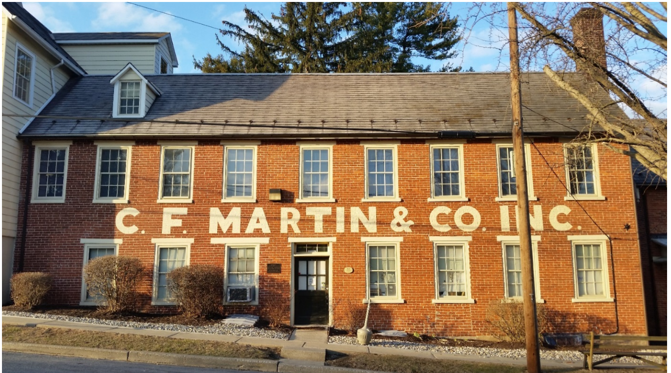
25. Front of Manufacturing Building 1. Camera facing north.
