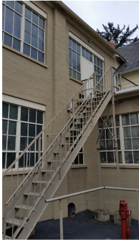
30. Staircase in front of Manufacturing Building 3. Camera facing northeast.
