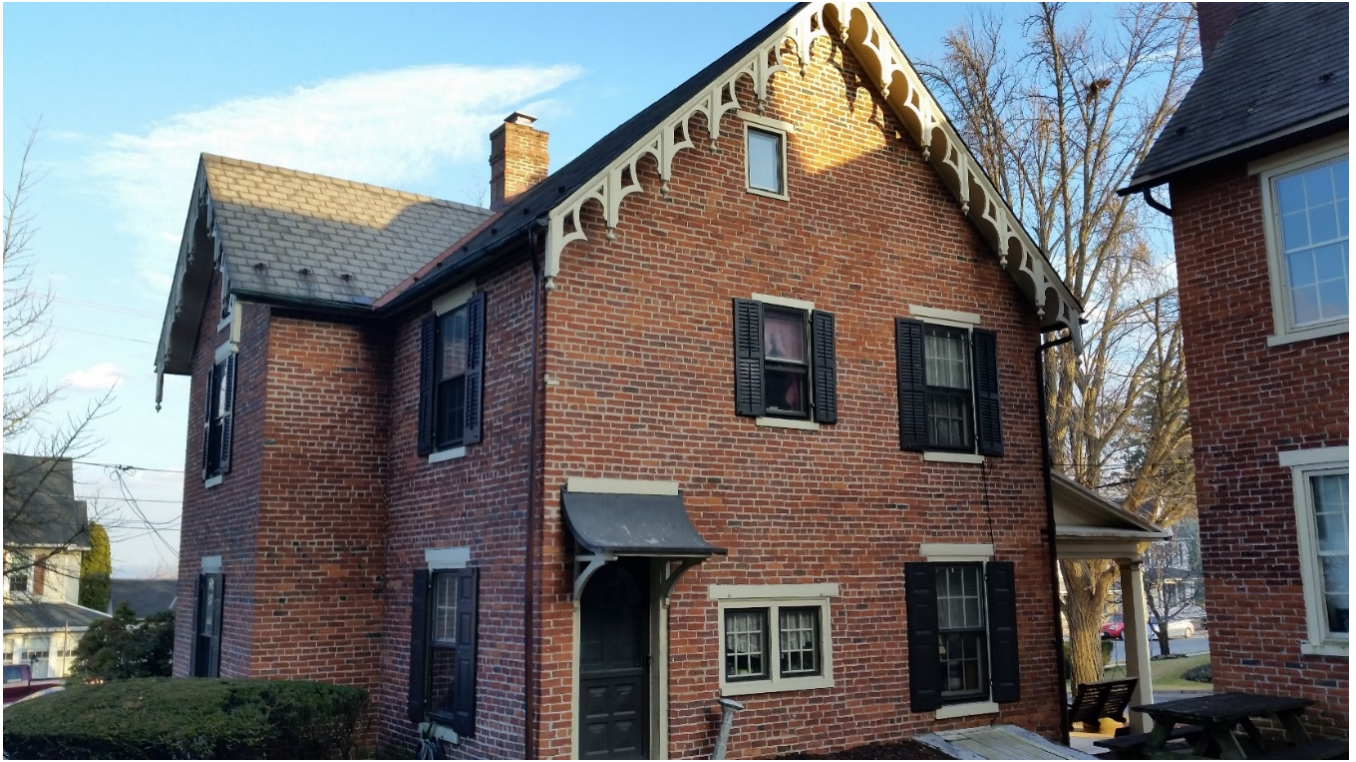
24. Back and side of the Martin House. Camera facing east.
