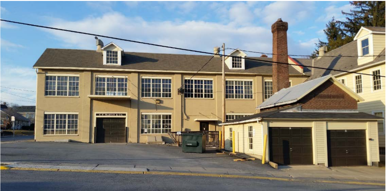
29. Front of Manufacturing Building 3 and Powerhouse. Camera facing north.
