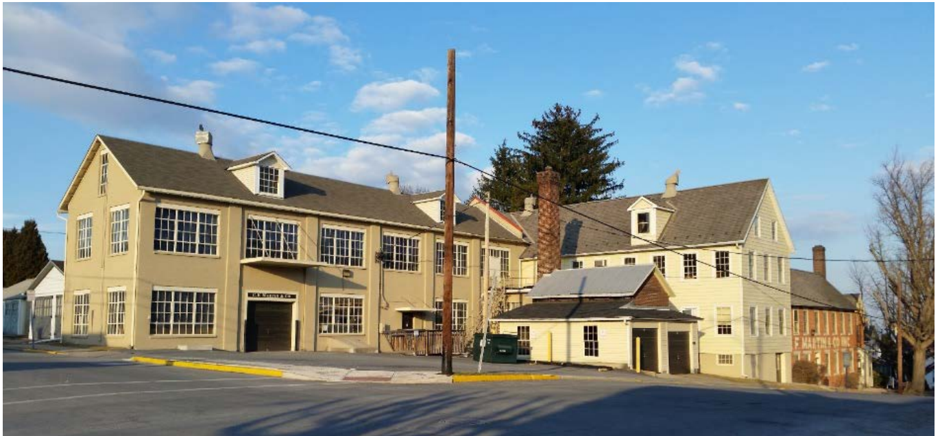
31. Manufacturing Buildings 1, 2, 3 and Powerhouse. Camera facing northeast.
