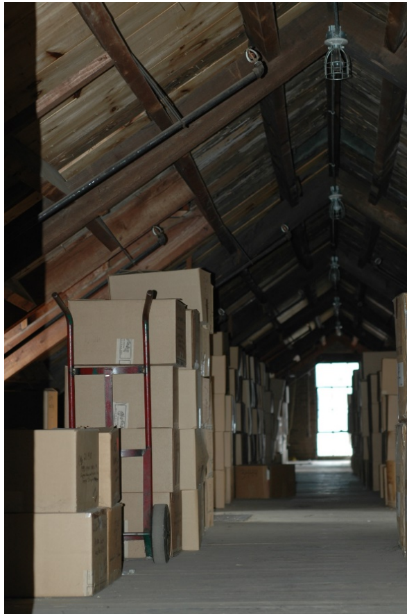
19. Manufacturing building 2 Attic used for storage. Camera facing south.
