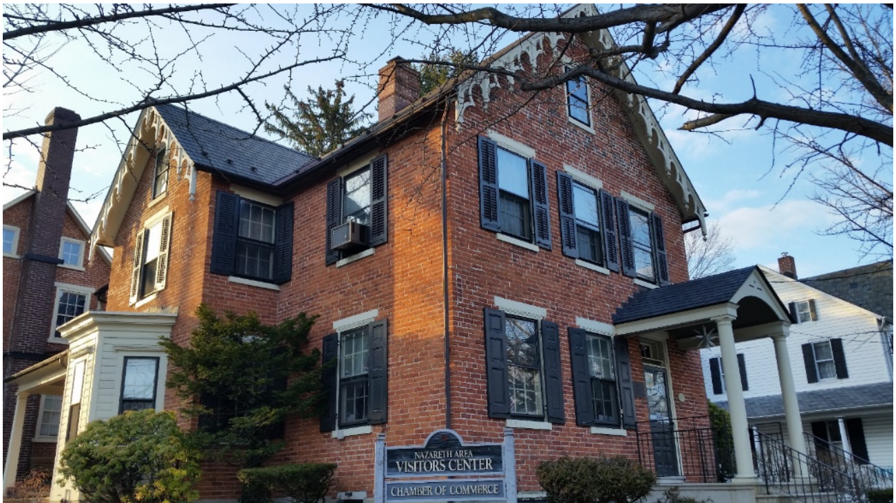
21. Front and side of the Martin House. Camera facing northeast.
