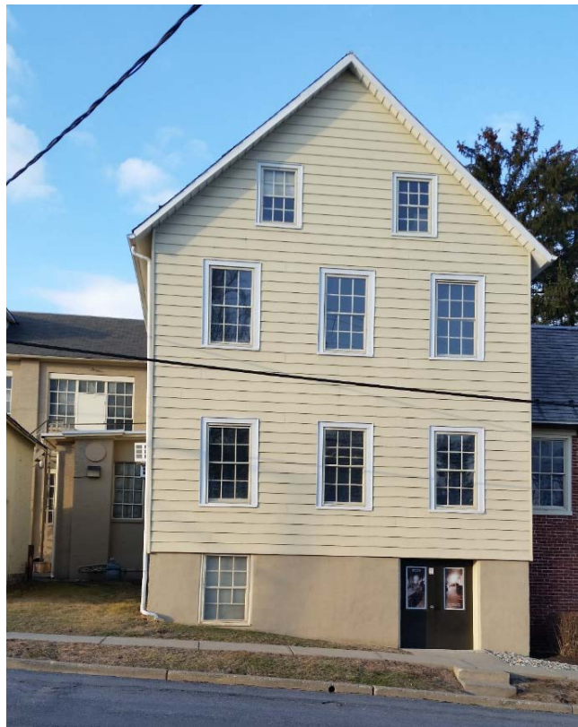
27. Front of Manufacturing Building 2. Camera facing north.
