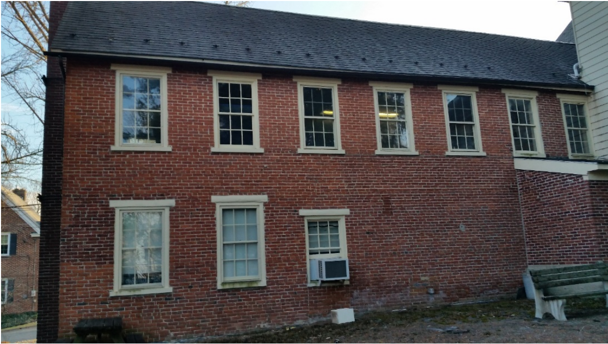
26. Back of Manufacturing Building 1. Camera facing south.
