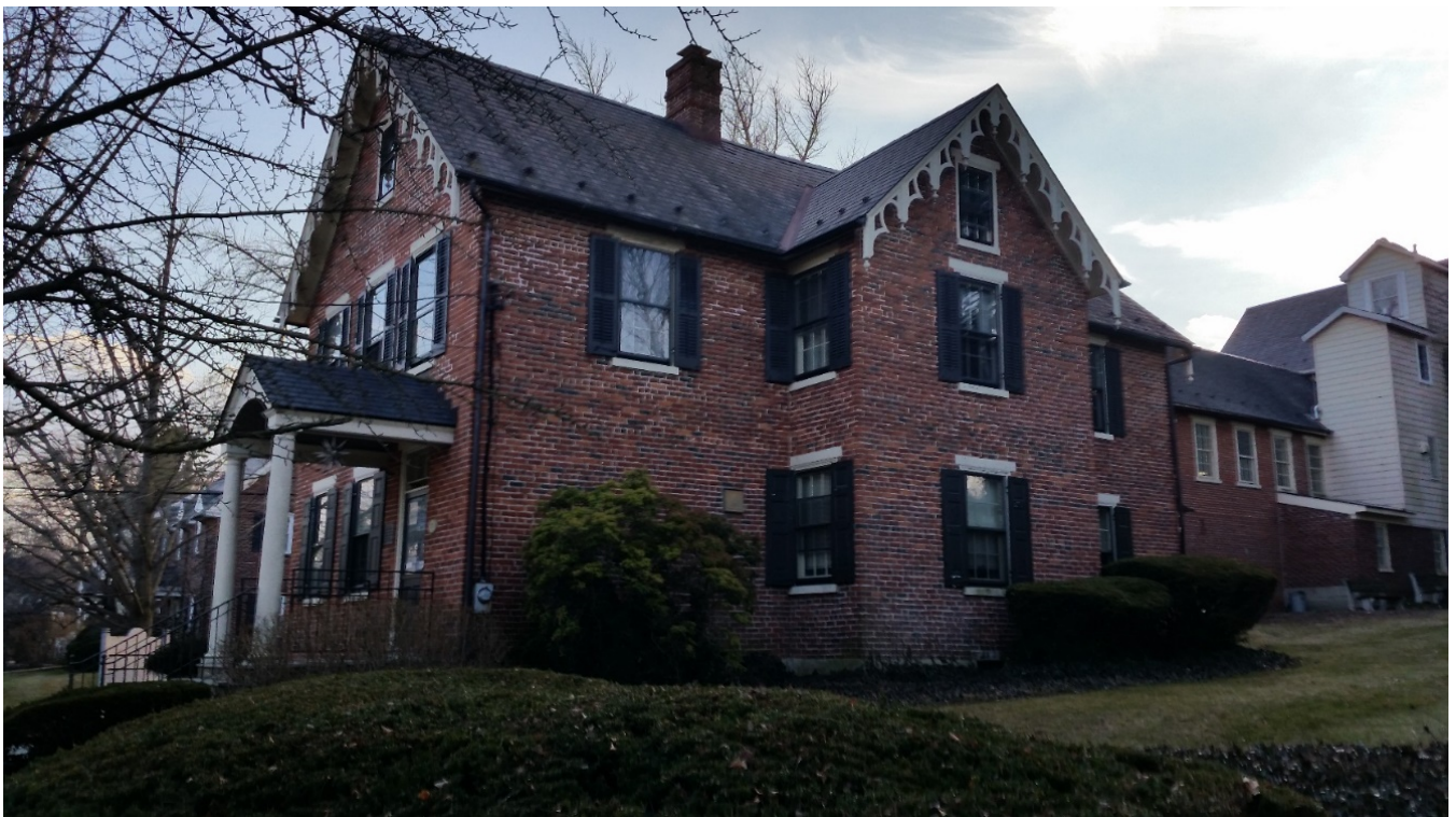
23. Front and side of the Martin House. Camera facing southwest.
