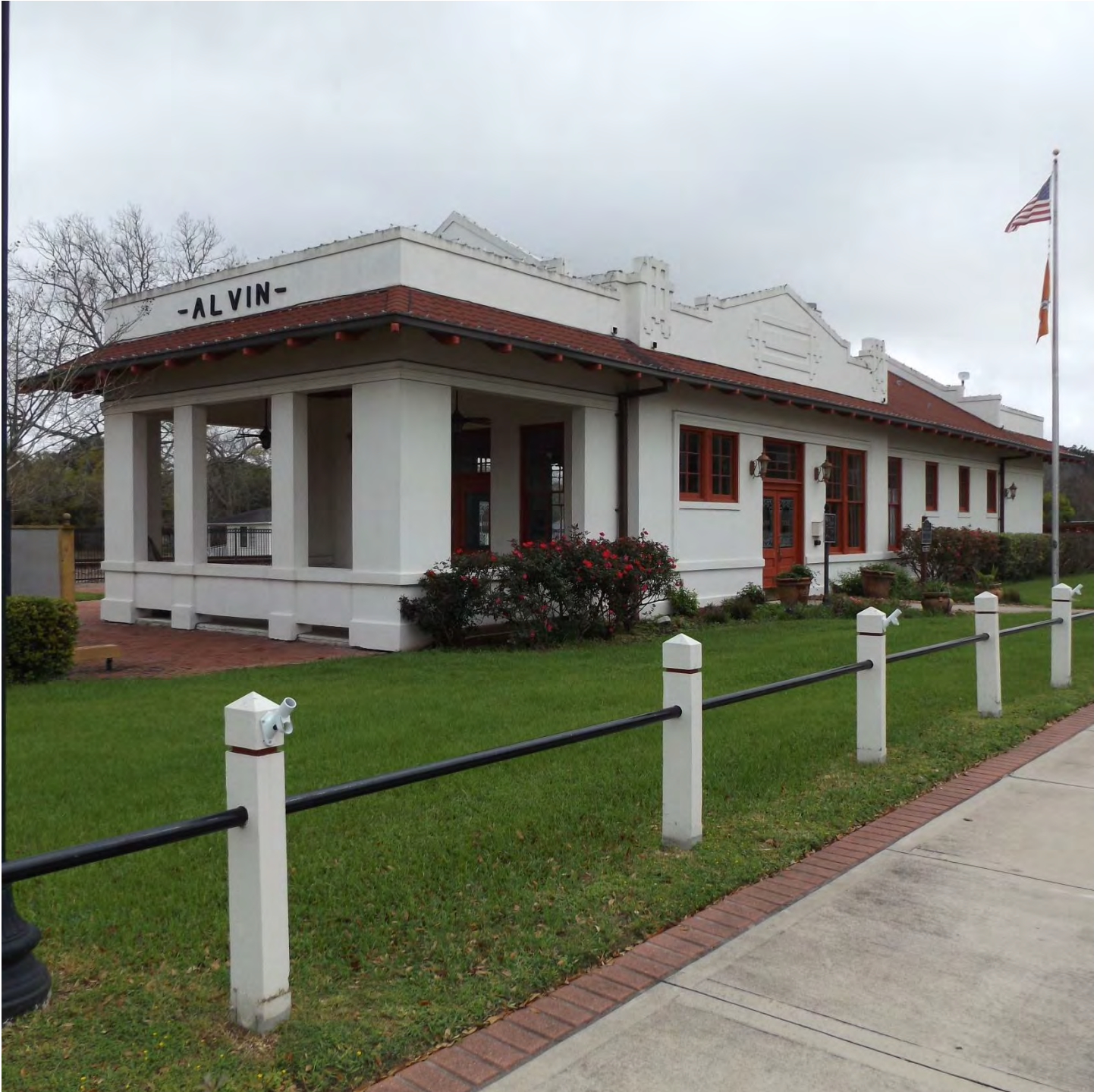
Photo 4 Oblique view of western and southern facades, facing northeast.
