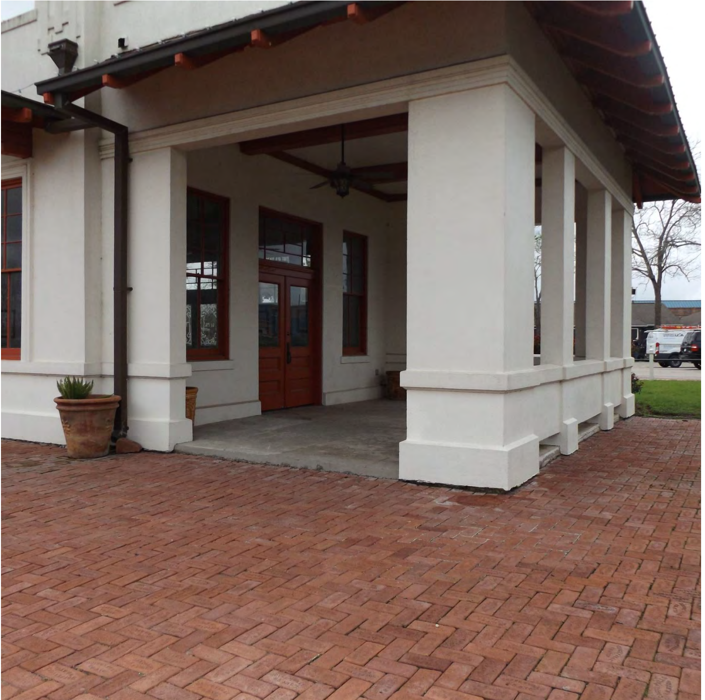
Photo 6 Detail of waiting room porch on west facade, facing southeast.
