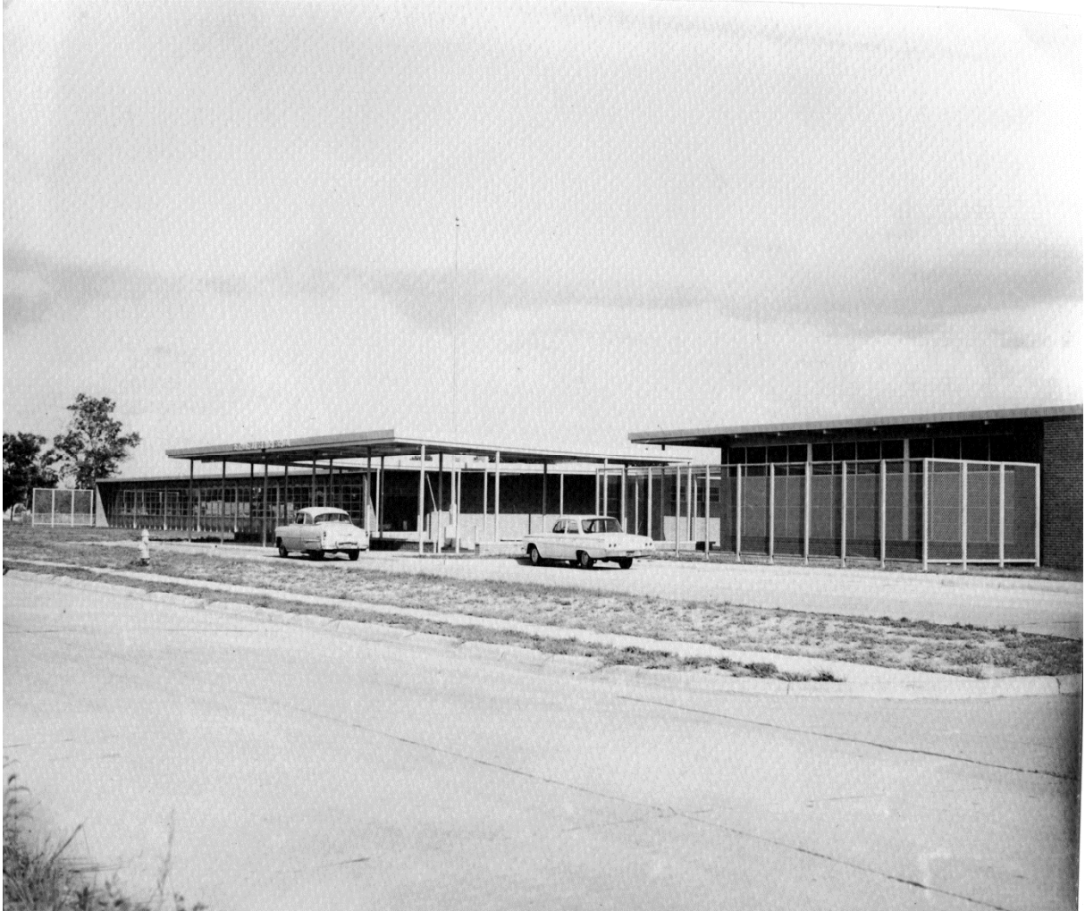
Figure 3: Bethune Jr-Sr High School front elevation from Henry Street before opening, 1961, Archives, Noel Library, LSU Shreveport
