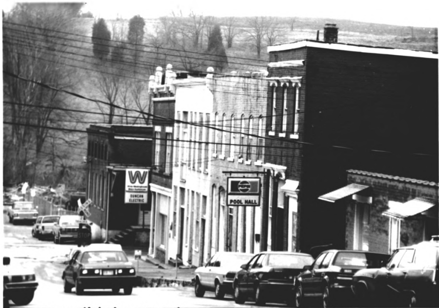
② Carlisle Historic District Nicholas County, KY
