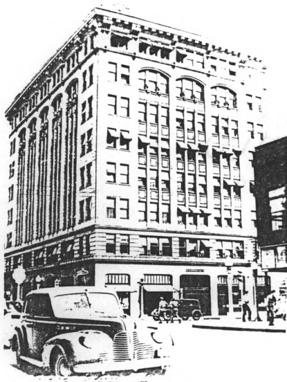
Modern Brotherhood of America (Brick & Tile Building) circa 1945. Looking southeast.
