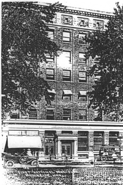
West elevation circa 1912. Note original location of main entrance in fourth bay from north.
