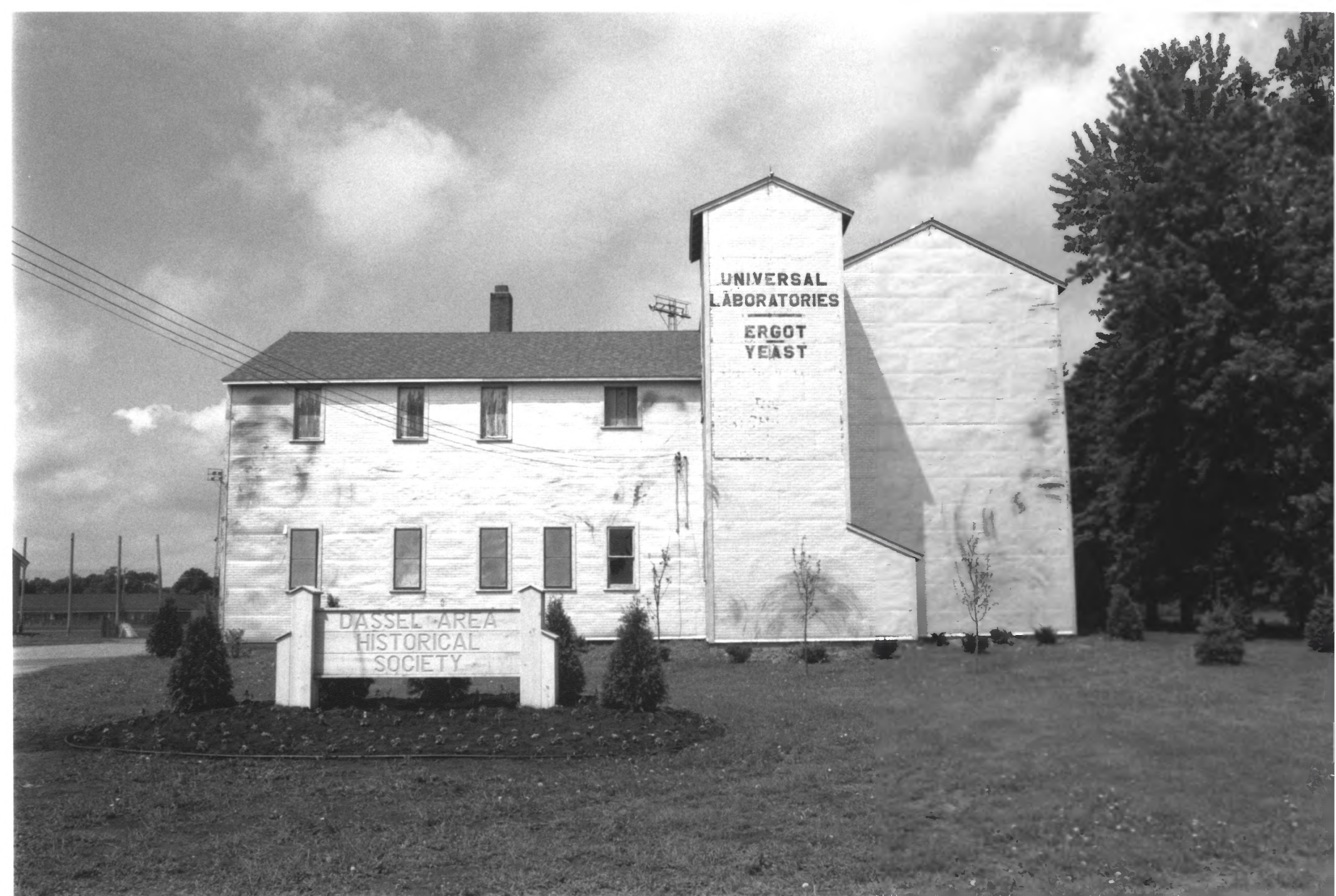
Universal Laboratories Building 901 First Street North, Dassel Meeker, Co., Mn 012570-7A18
