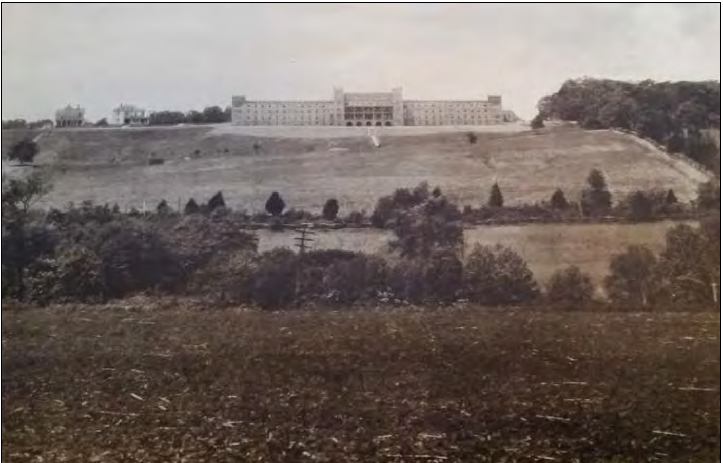
Figure 5: Tennessee Military Institute main building from the east. 1311 and 1313 Peachtree Street are visible, c.1910. Source: TMI Catalog, 1915 (McClung Archives, East Tennessee History Center).
