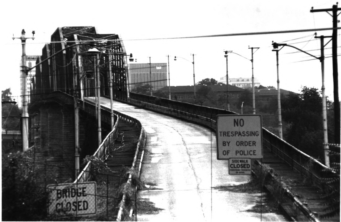
WALNUT STREET BRIDGE HAMILTON COUNTY TN
