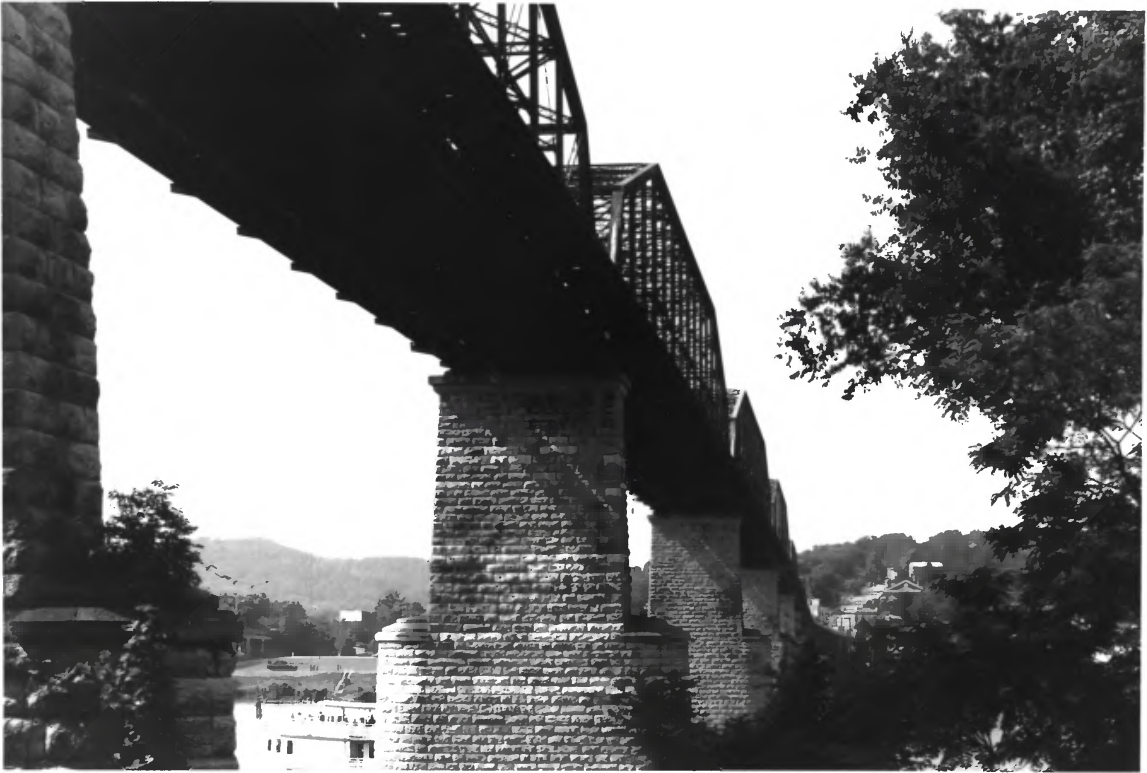
WALNUT STREET BRIDGE HAMILTON COUNTY TN
