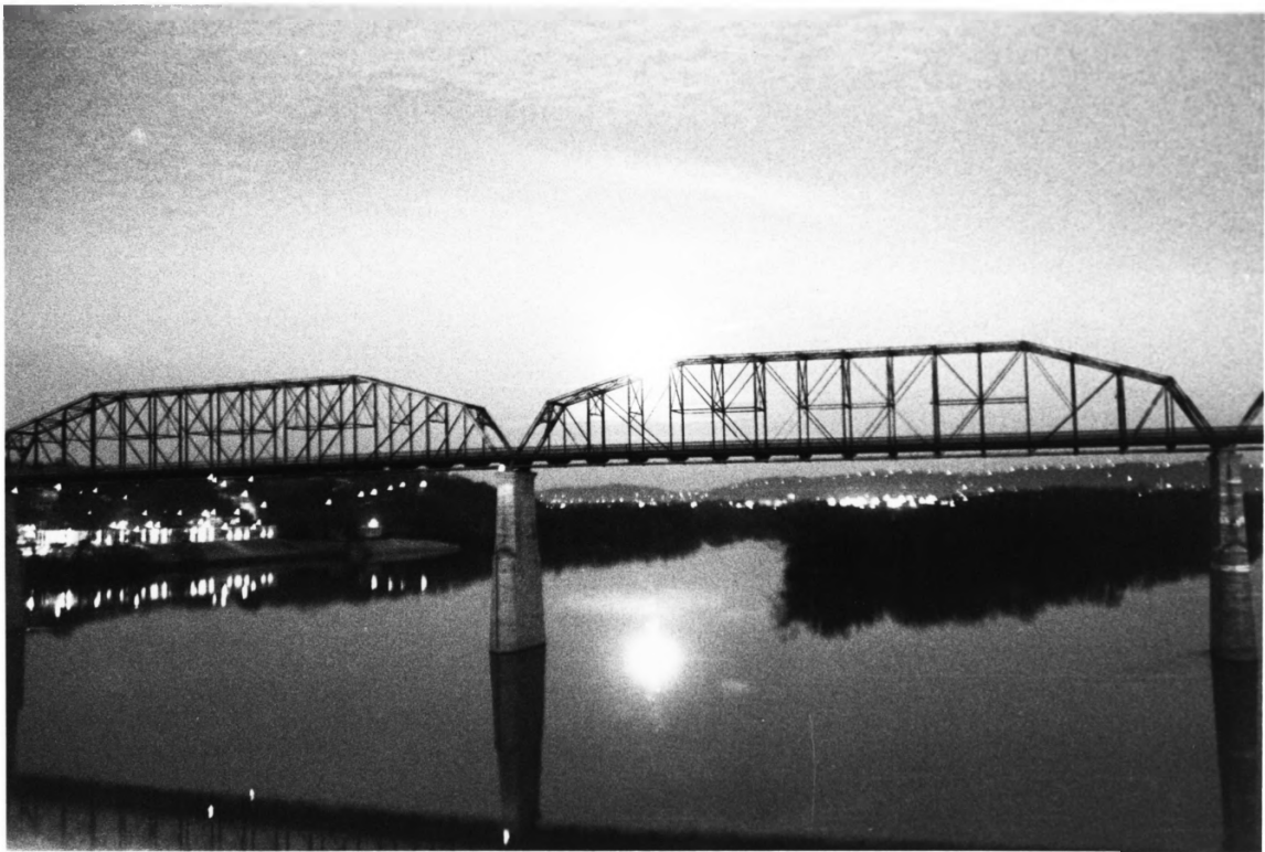
WALNUT STREET BRIDGE HAMILTON COUNTY TN
