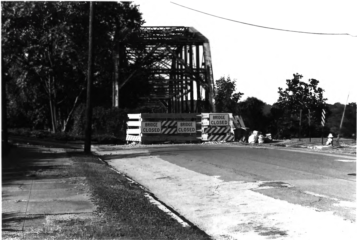
WALNUT STREET BRIDGE HAMILTON COUNTY TN
