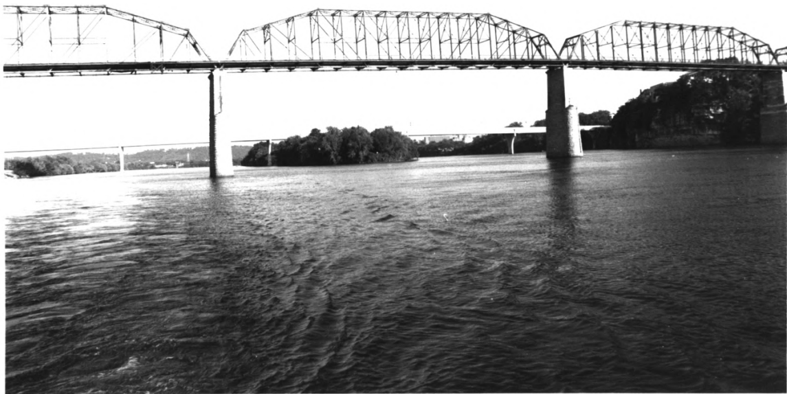
WALNUT STREET BRIDGE HAMILTON COUNTY TN
