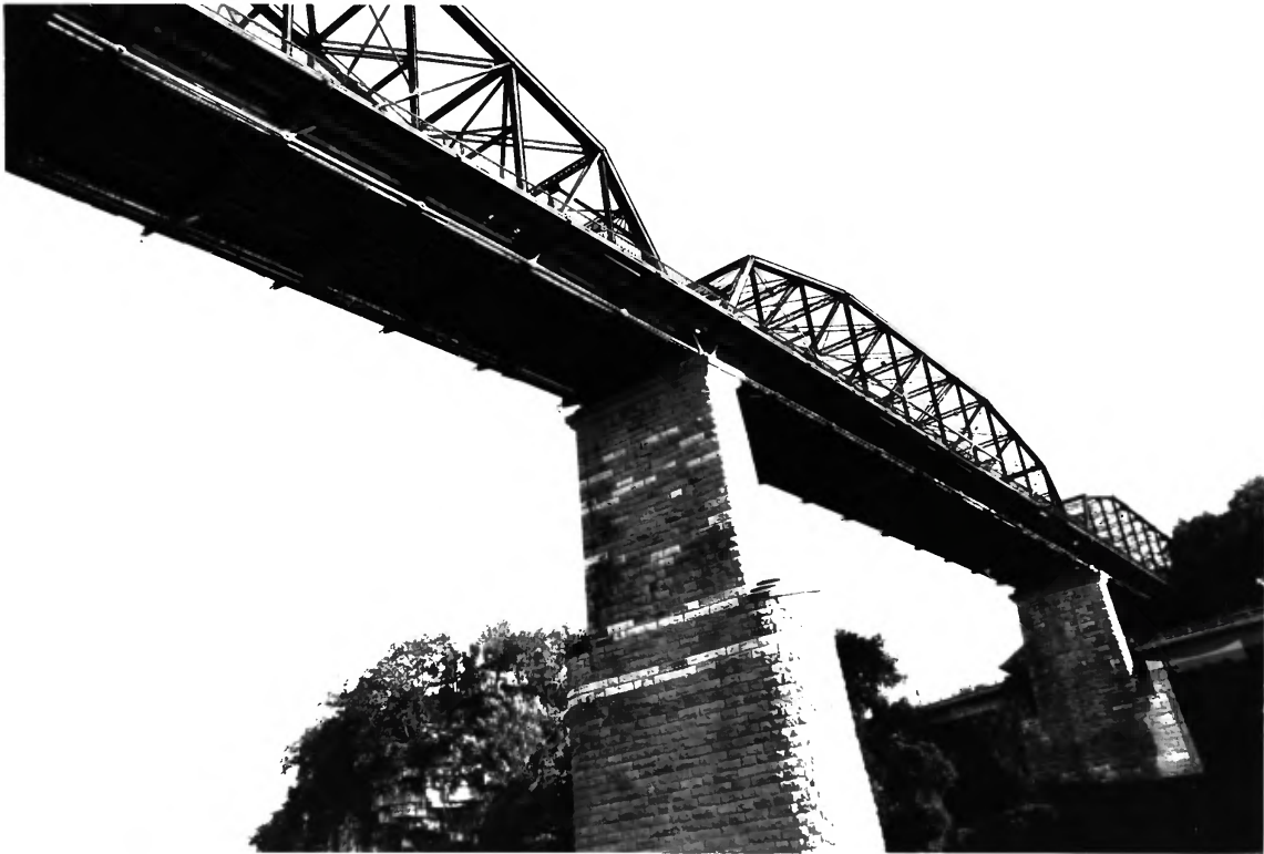
WALNUT STREET BRIDGE HAMILTON COUNTY TN
