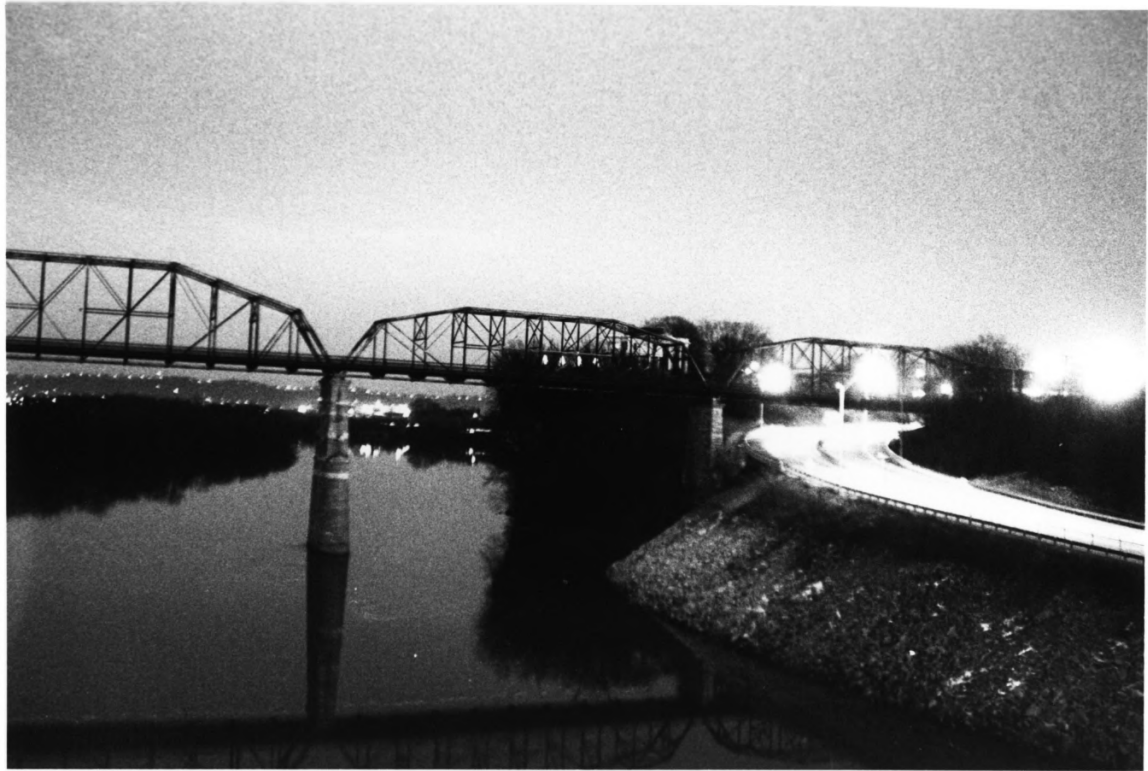
WALNUT STREET BRIDGE HAMILTON COUNTY TN
