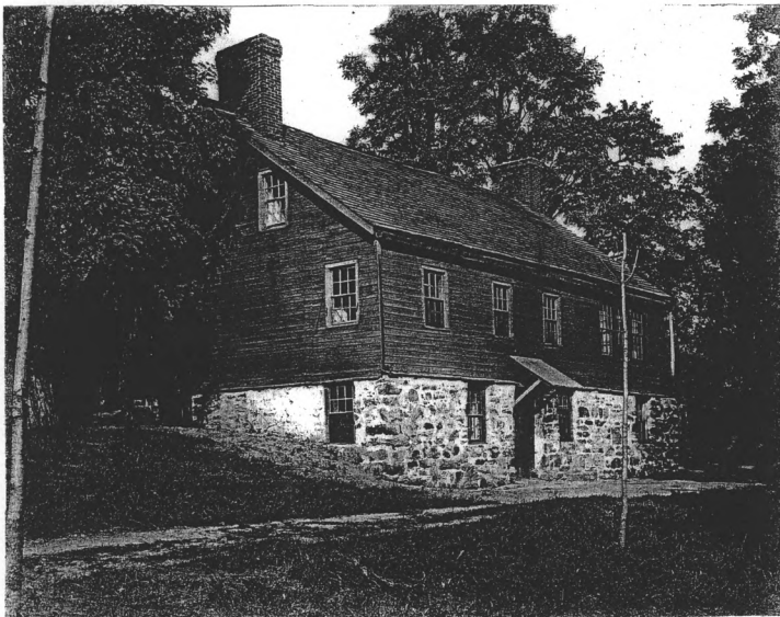
Luke Miller House, 105 Ridgedale Avenue, prior to restoration and expansion. (Photograph courtesy of the Madison Historical Society)
