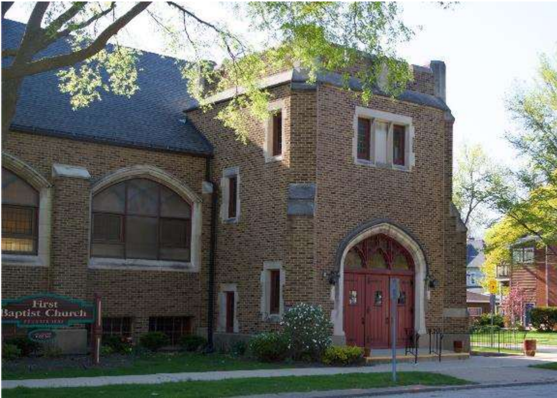
Figure 43: Comparison, First Baptist Church, 20 North Ashland Avenue, La Grange
