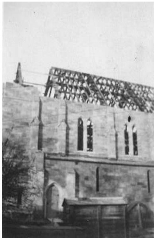
Figure 30: View of south façade, December 1925
