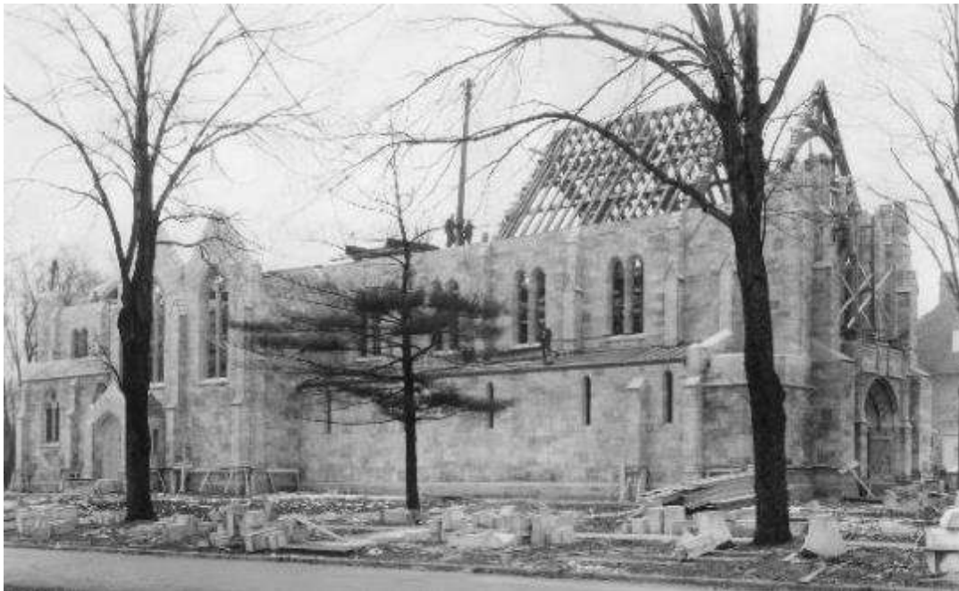
Figure 26: View of north façade from the northwest, December 1925
