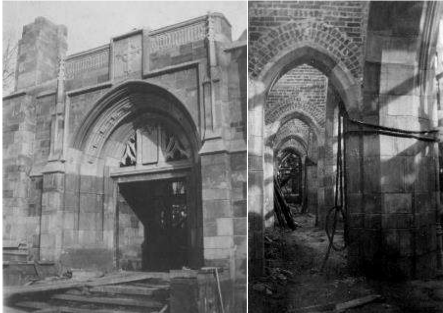
Figure 21 (left): View of west entrance from southwest, November 1925
