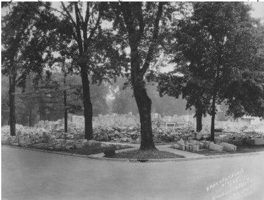
Figure 14: Starting the stone walls, August 3, 1925
