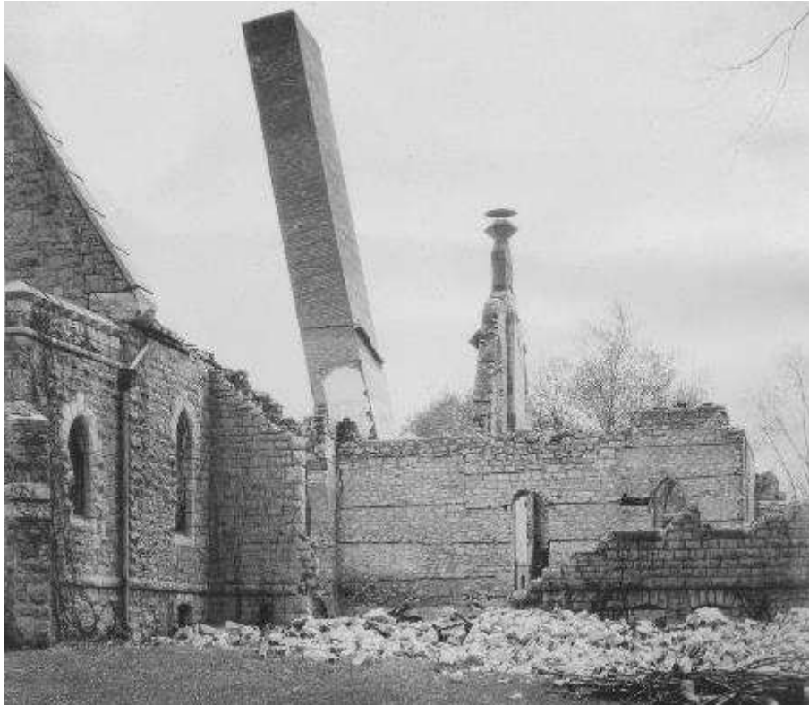
Figure 13: Dynamiting the chimney and clearing the ruins of the old church from the site, April 25, 1925
