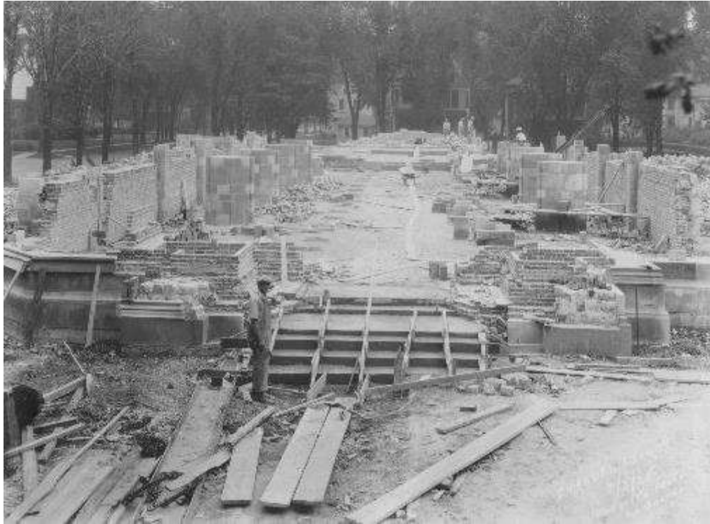
Figure 15: View from west showing the beginnings of raising the brick backed stone walls and stone columns in the church interior, August 3, 1925
