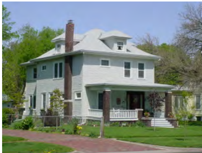
American Foursquare at 1335 N. Broad
