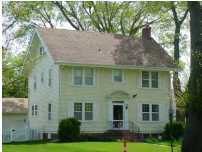
Colonial Revival House at 1210 North Broad Street
