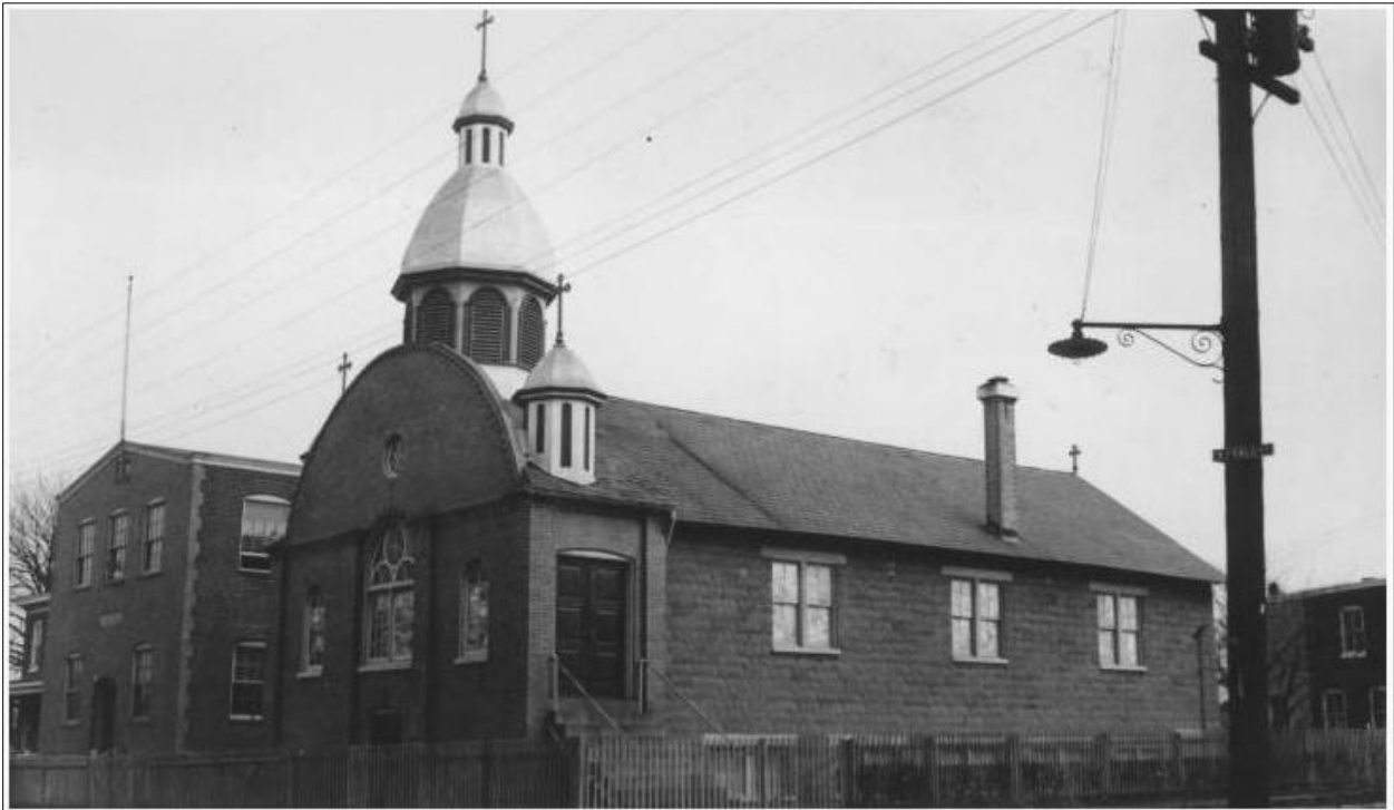
Figure 7: St. Nicholas Ukrainian Catholic Church, view of northwest and southwest elevations, 1936. Delaware Public Archives, Frank R. Zebley Collection, Churches of Delaware Photograph Collection, no. RG 9015-001-002.
