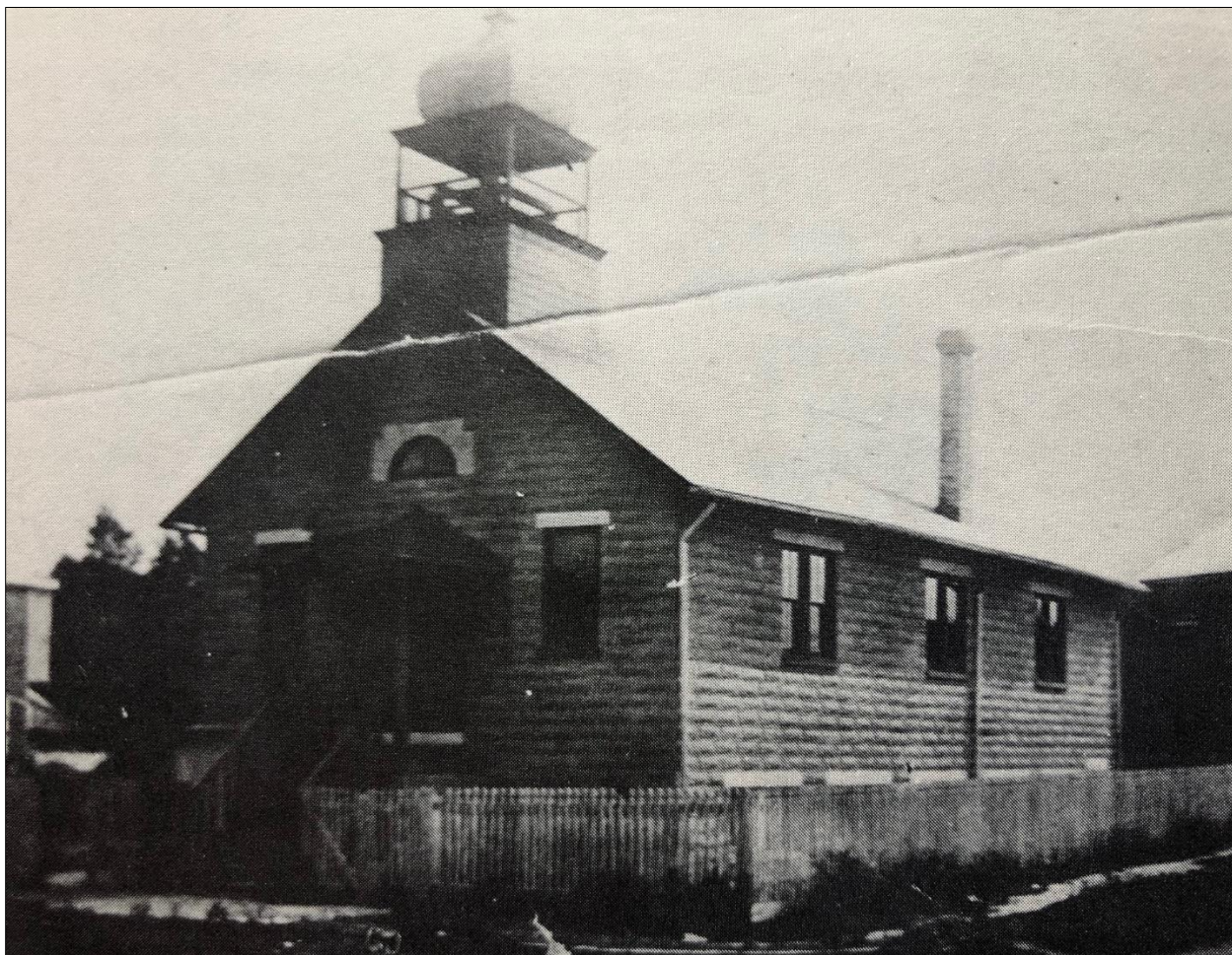
Figure 5: St. Michael's United Greek Catholic Ruthenian Church, later St. Nicholas Ukrainian Catholic Church, view of northwest and southwest elevations as originally constructed, 1909. From Lushnycky, 75 Jubilee , 115.
