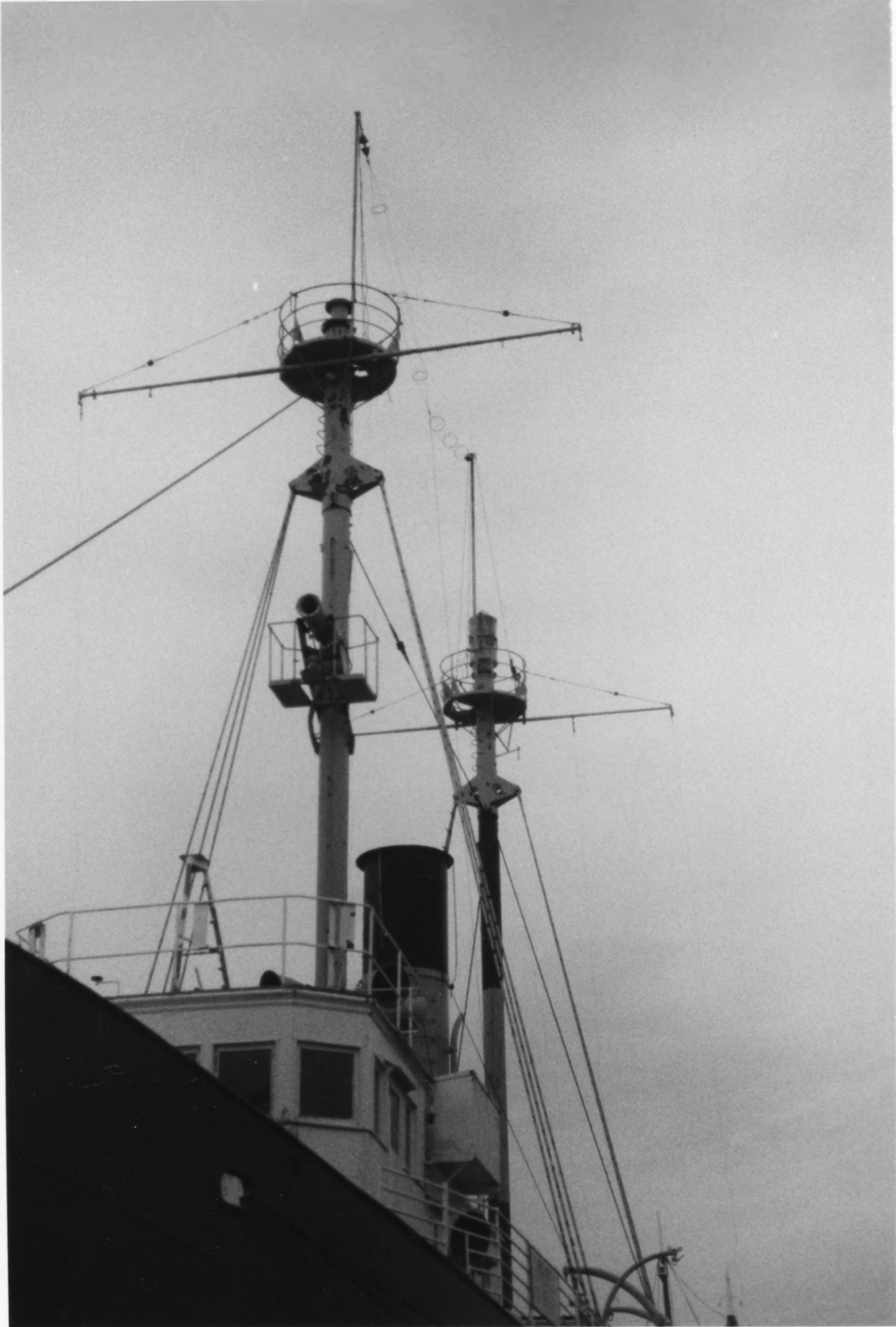
LIGHTSHIP NO. 83, Kirkland, Washington Photo by James P. Delgado, 1988 (NPS) Northwest Seaport, Inc. Masts and lights, Photo #4
