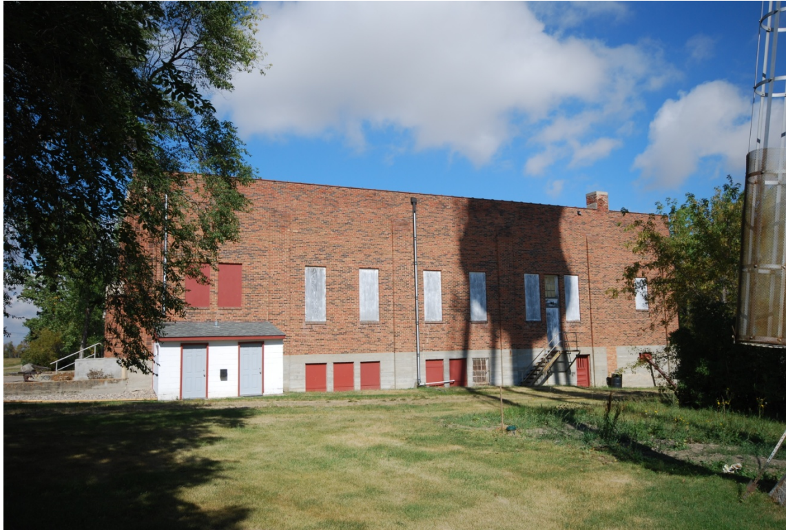
6 of 6, Southeast side
