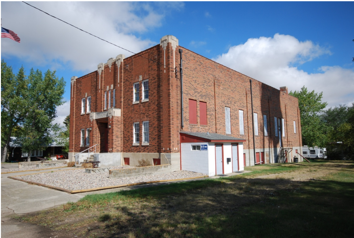
5 of 6, South corner
