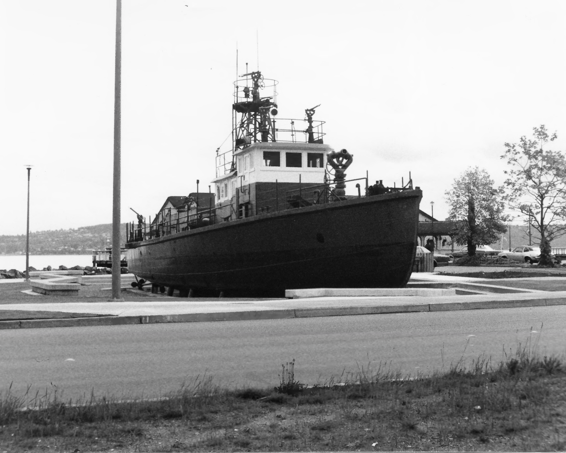
FIREBOAT NO. 1, Tacoma, Washington Photo by Allen Ratcliffe, 1988 Tacoma Fire Department View, starboard bow. Photo #6
