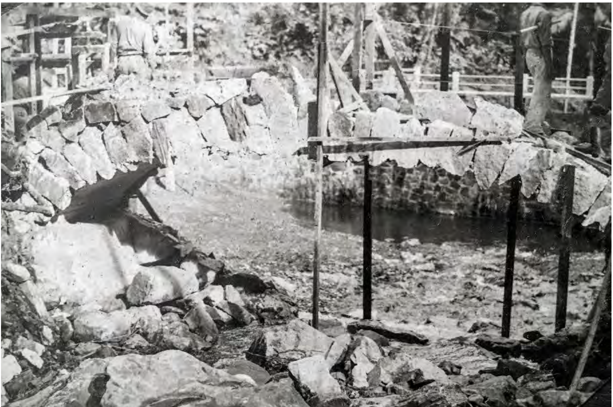
Figure 21. Construction of concrete arched bridge (1938) (EYNF Heritage Program Records).
