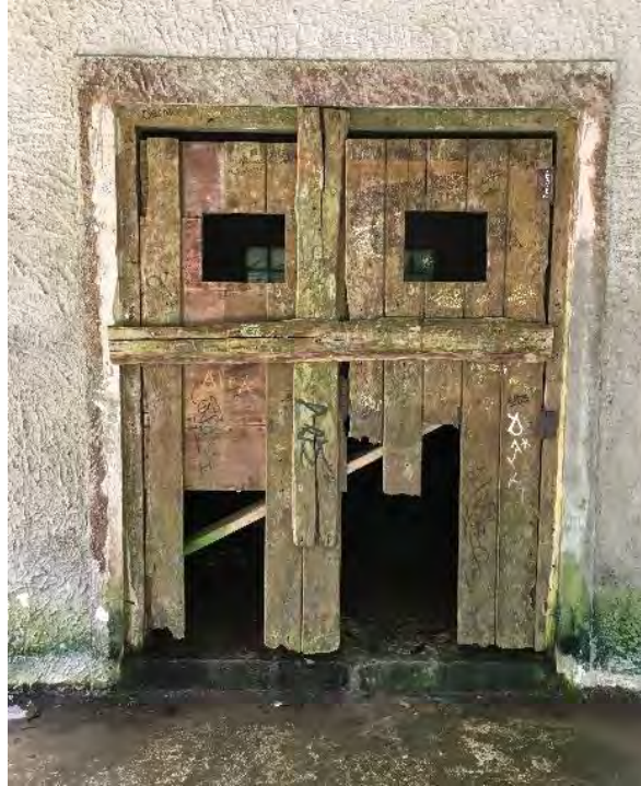
Figure 14. View of central doorway (towards the south).
