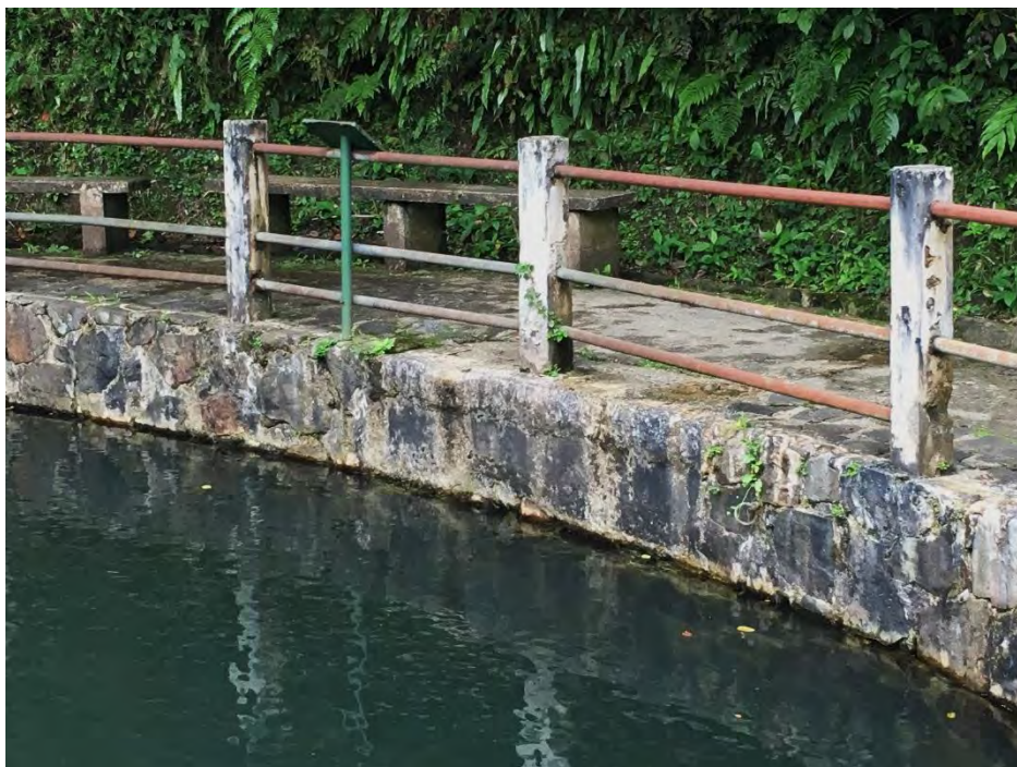
Figure 9. View of railing extending around the pool's edge (towards the northwest).
