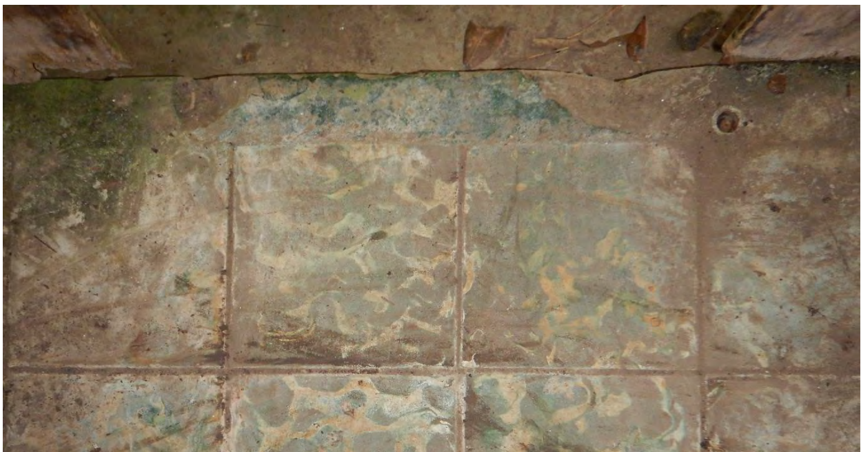
Figure 24. Original tiles behind the bathhouse entrance doorway.
