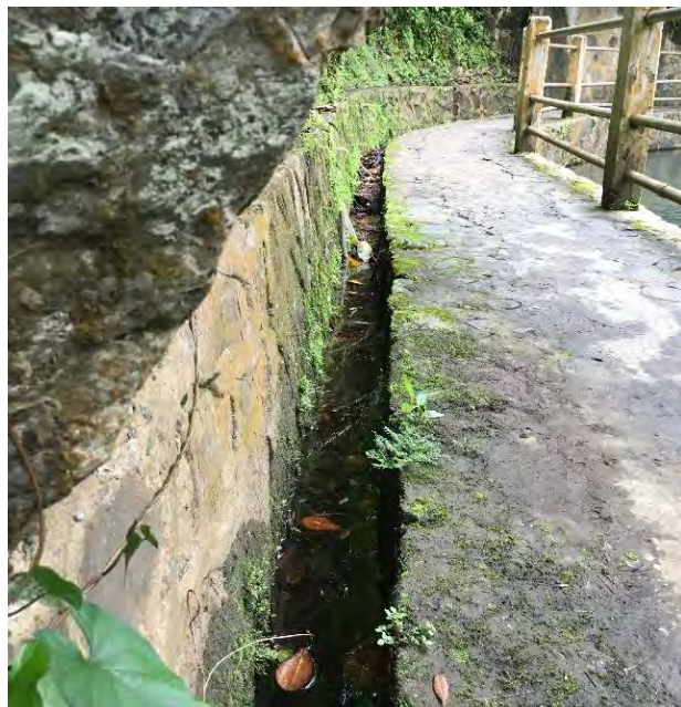
Figure 7. View of southern walkway drainage (towards the southwest).
