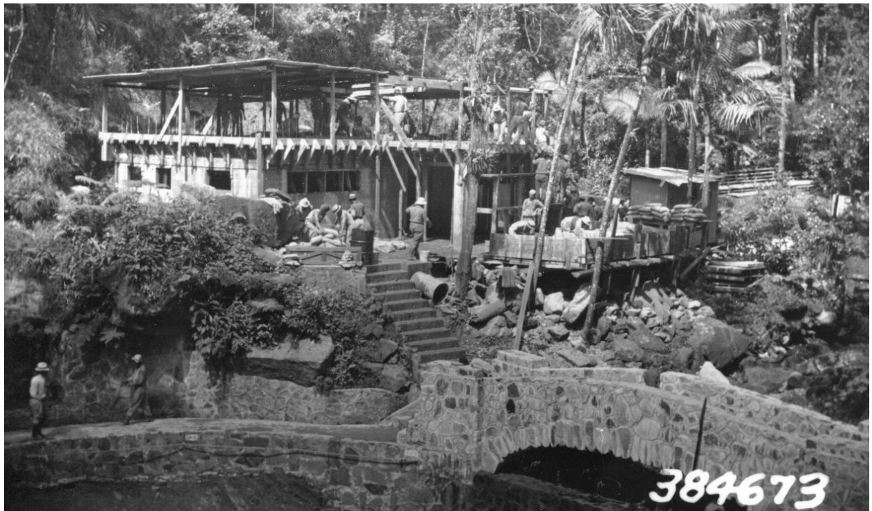
Figure 23. Construction of the concrete bathhouse (1938) (EYNF Heritage Program Records).
