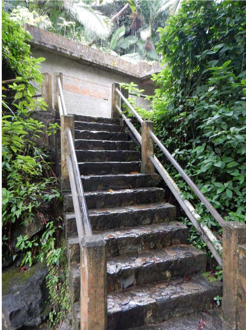
Figure 13. Bathhouse access stairway (towards the south).
