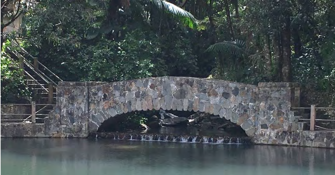
Figure 11. View of the concrete arched bridge (towards the west).
