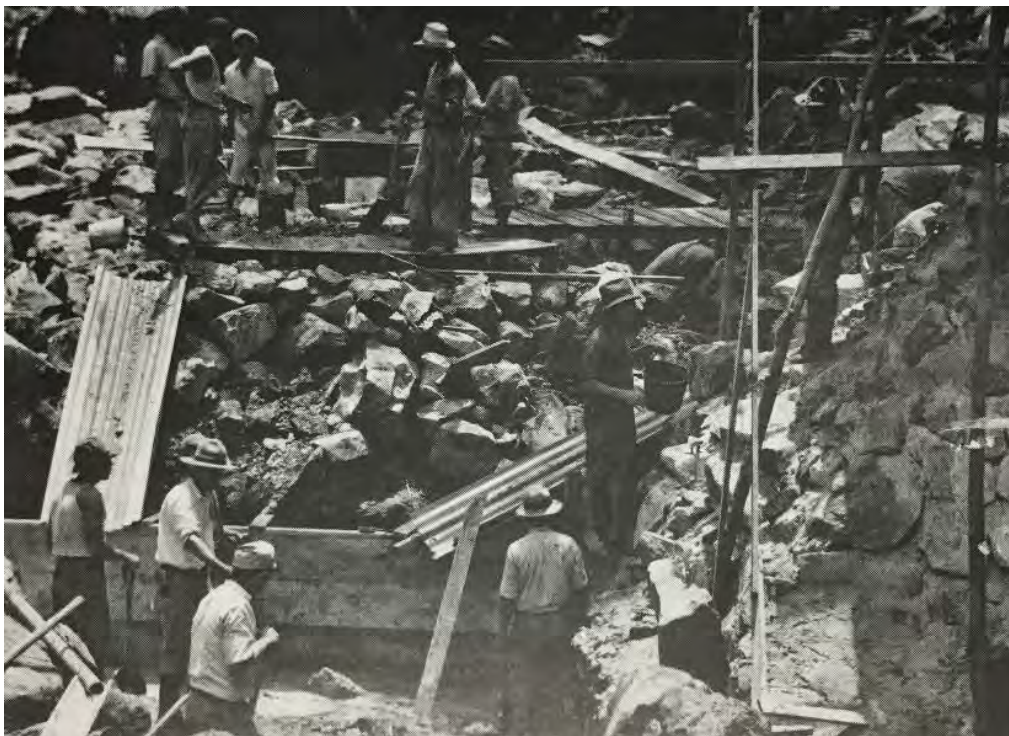
Figure 18. Construction of Baño Grande dam (1936) (EYNF Heritage Program Records).
