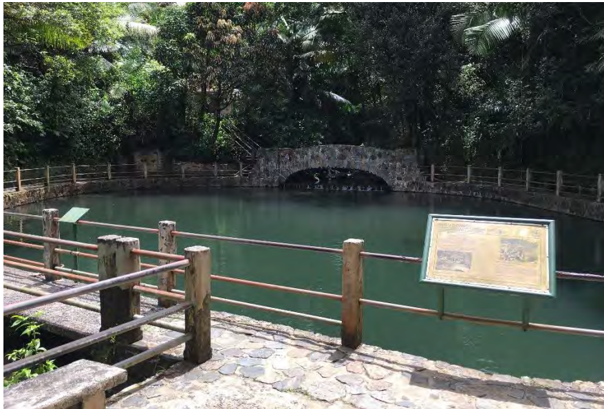
Figure 4. General view of the pool (towards the southwest).
