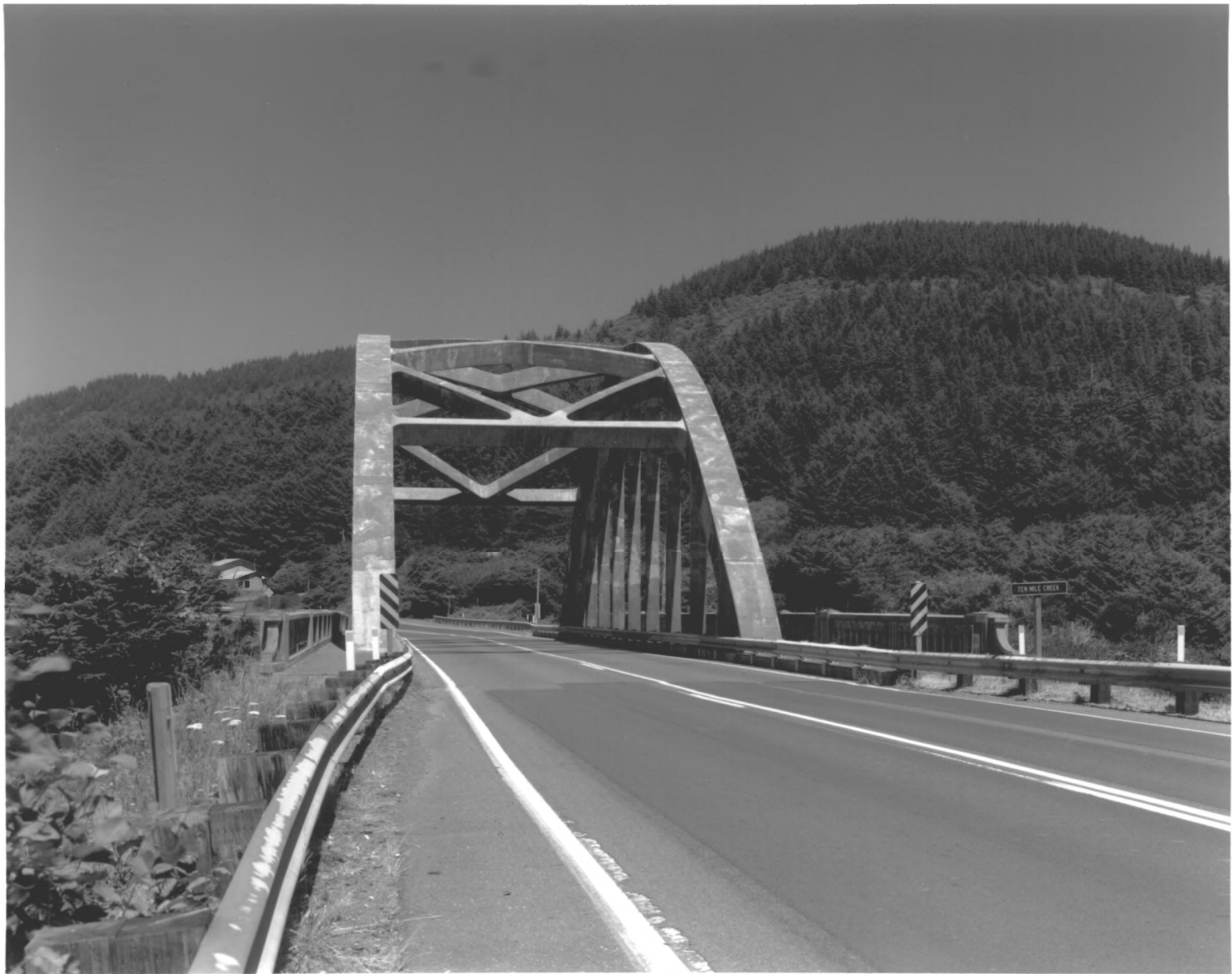
TENMILE CREEK BRIDGE, YACHTS VICINITY, OREGON #1
