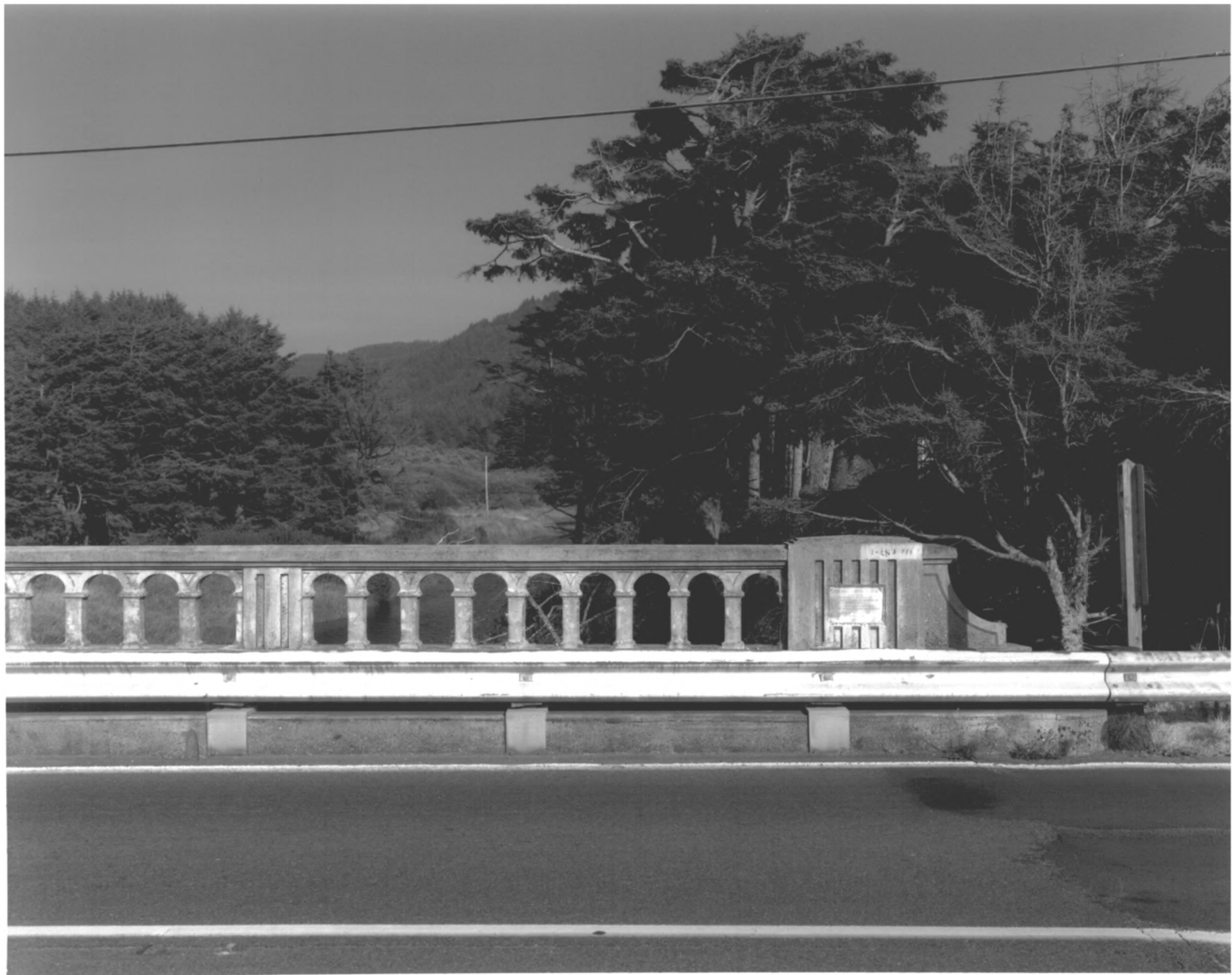
TEN MILE CREEK BRIDGE, YACHTS VICINITY, OREGON # 5
