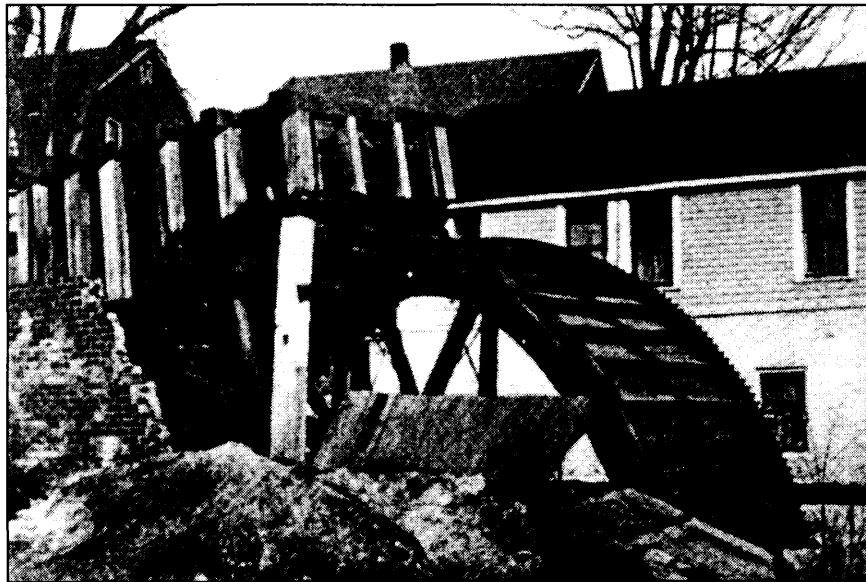
Figure 3: Terryville Waterwheel in 1951 (Harte 1956). The partial brick wall is a remnant of the brick basement story of the mill.
