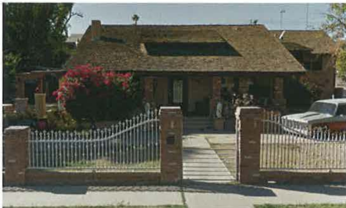
House at 456 N. Robson St., prior to rehabilitation of porch posts. Source: Google, 2016.
