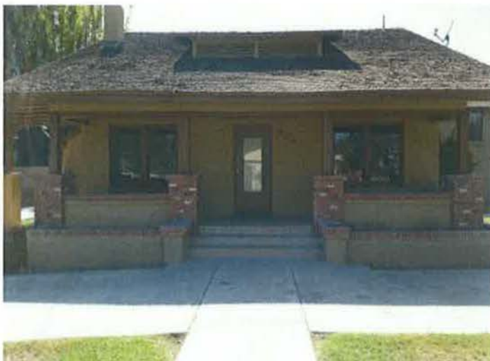
House at 456 N. Robson St., after rehabilitation of porch posts. Source: Lauren Allsopp, City of Mesa Historic Preservation Office, 2018.
