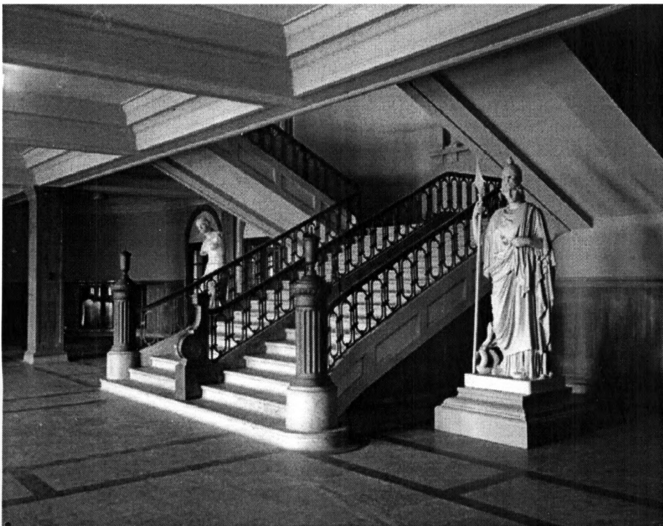
Figure 2. Circa 1925 view of the main stair rising from the first-floor lobby. Source: Western History/ Genealogy Department, Denver Public Library
