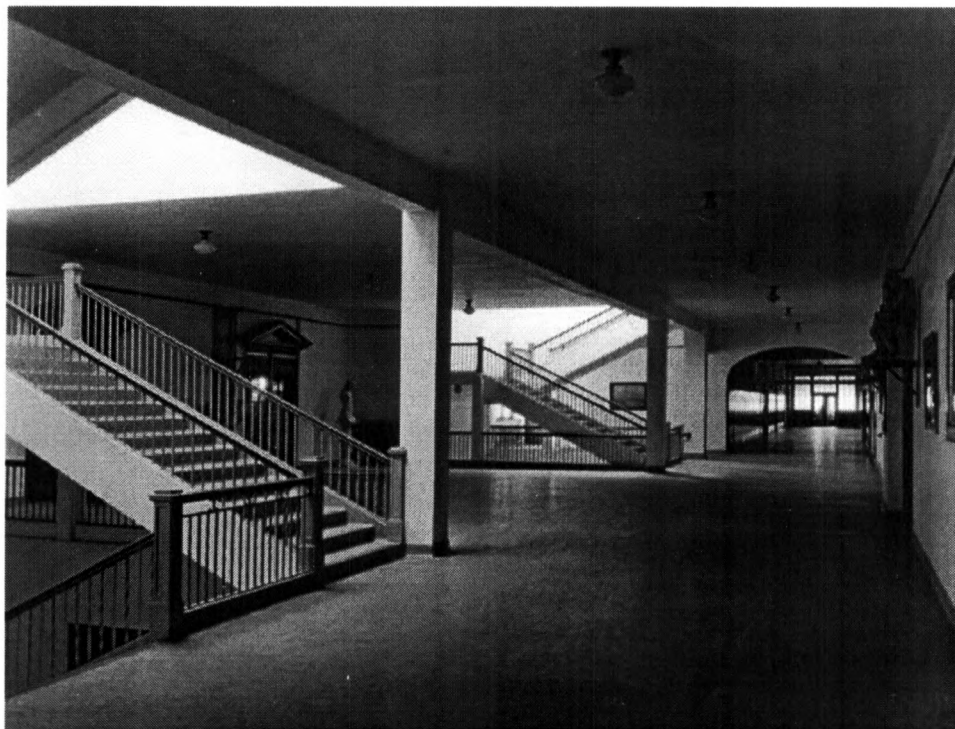
Figure 3. Circa 1925 view of the main stair and the third-floor hallway.
