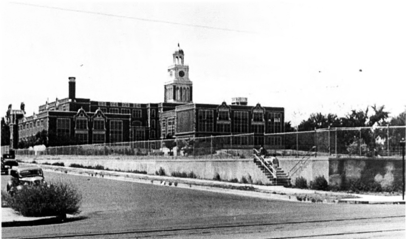
Figure 8. This 1936 view of East High School shows the north side of the building prior to the construction of the gymnasium addition.
