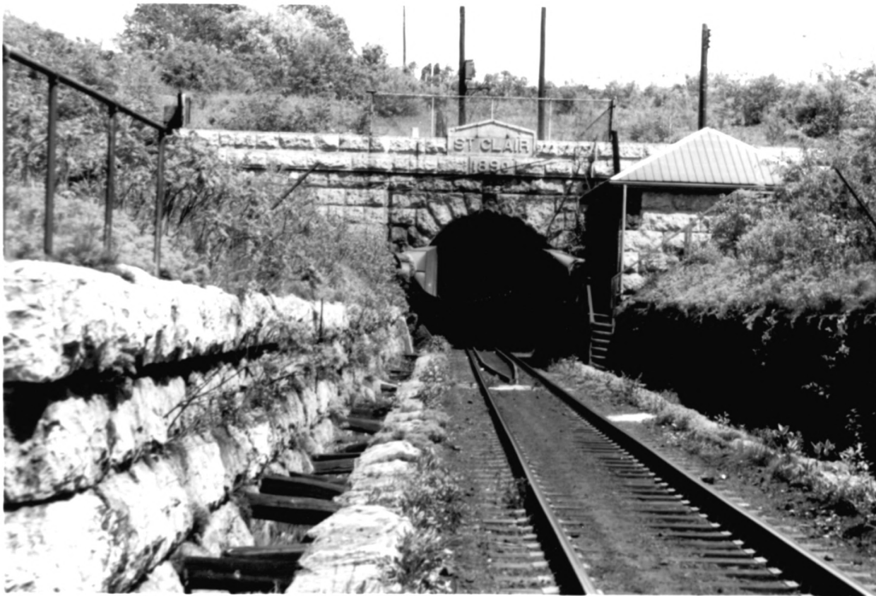
PHOTOGRAPH #1 St. Clair River Tunnel Port Huron, Michigan Port Huron Portal, Looking East Robie Lange, 1992
