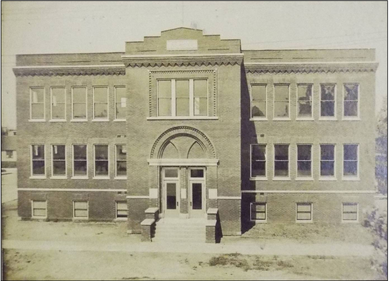
Appendix D - 1914 school building soon after its completion. The photo reveals a detail not evident on the structure today; the second floor window located directly above the main entry. This opening has been filled with glass block and brick. Photograph in St. John's Church archives.
