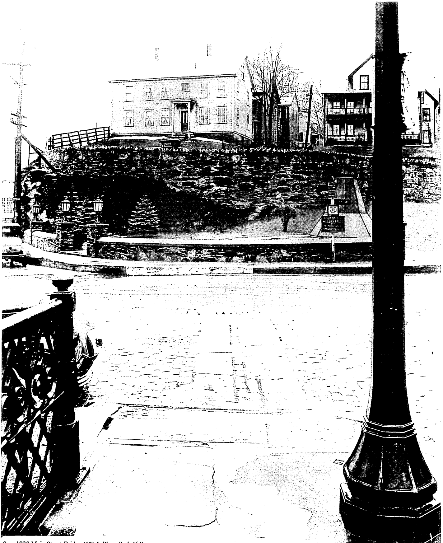
9. c. 1930 Main Street Bridge (63) & Plaza Park (64), Brattleboro Downtown Historic District (Boundary Increase), Brattleboro, Windham Co., Vermont, Courtesy Brattleboro Historical Society
