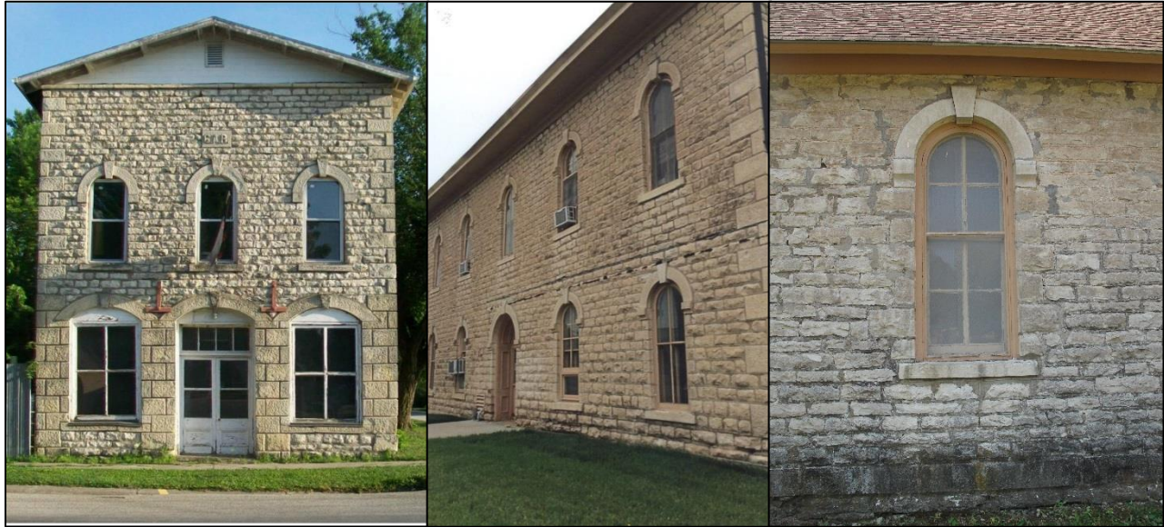
Figure 3: At left, G.A.R. Building (c. 1885); Center, Pottawatomie County Courthouse (1884); Right, Window Detail of German Evangelical Church (1887). All photos from the KHRI.
