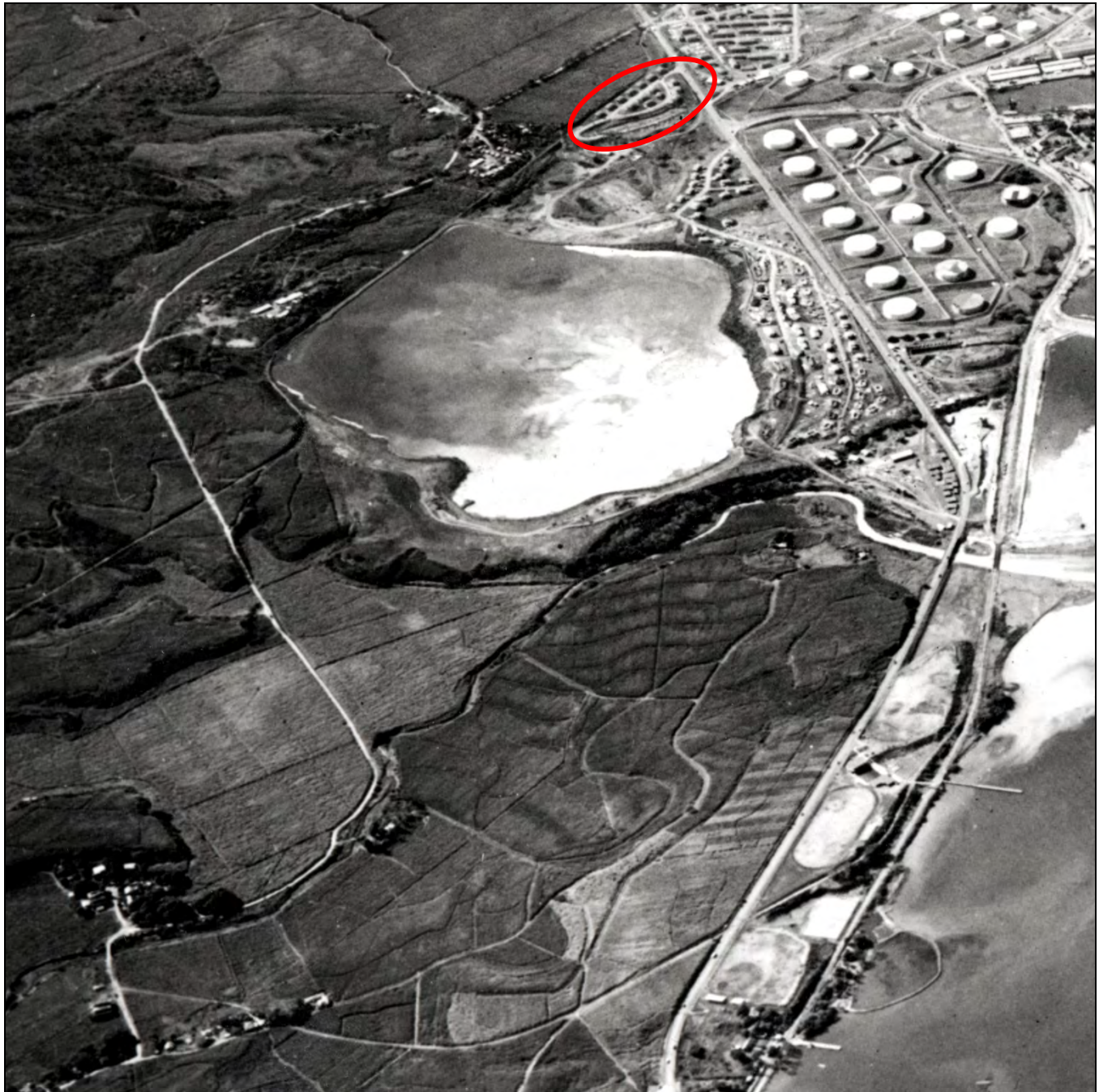
Figure 8-10. Aerial photograph dated November 1941, showing the Little Makalapa Naval Housing Historic District under construction, circled in red. All 15 duplex units are visible. Source: National Archives, College Park, Maryland, Still Pictures Collection, Record Group 30, Photo No. 80-G-182874.
