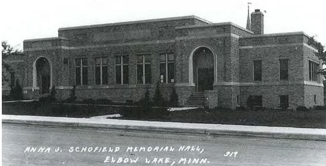
Figure 14: Building in 1934. Photo provided by Grant County Historical Society.
