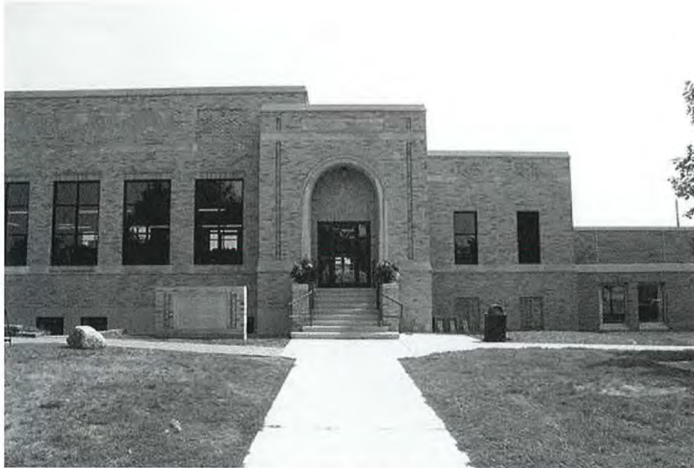
Figure 1: West facade with 1977 addition on the far right. Camera facing east.
