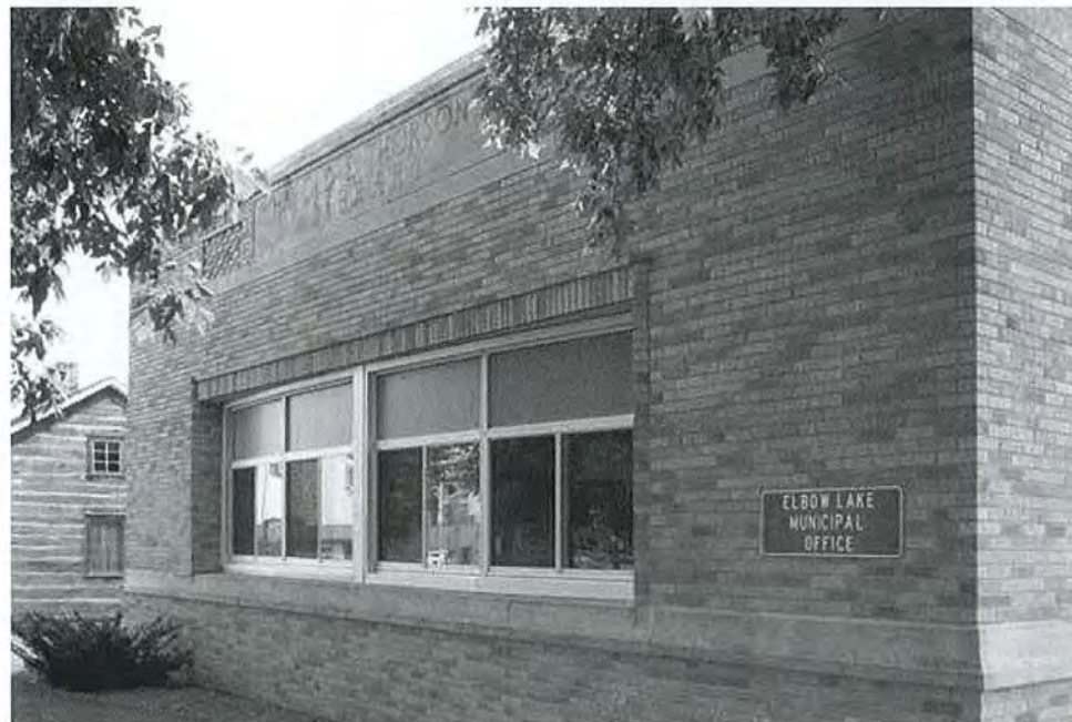
Figure 4: Window on north elevation. Camera facing southeast.
