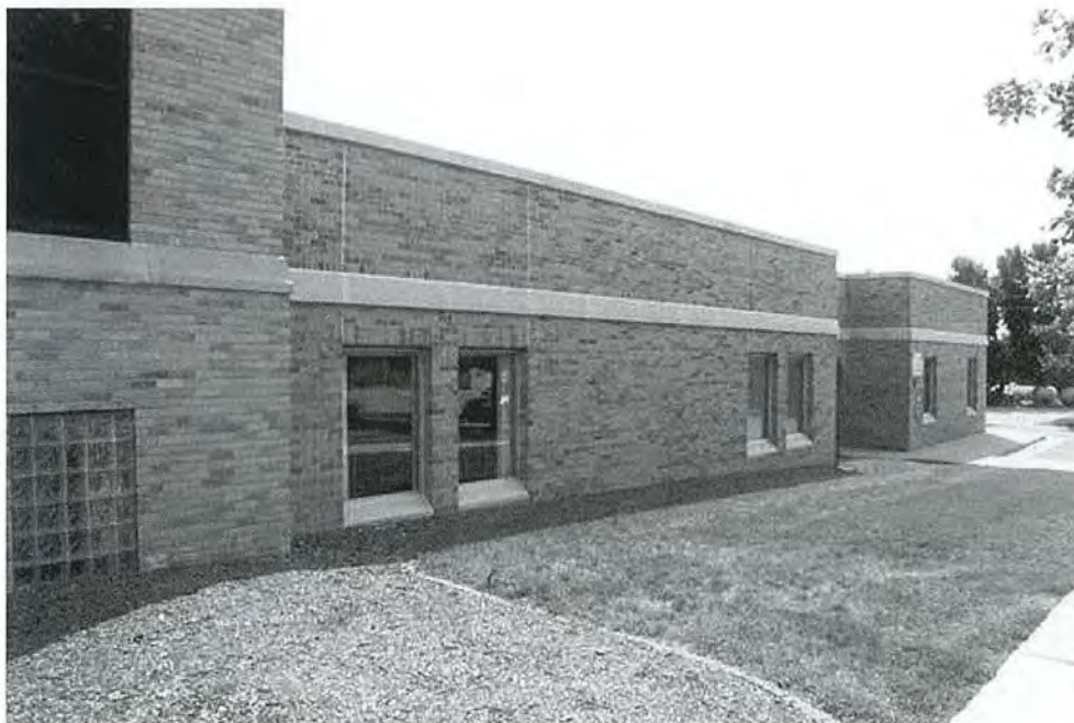
Figure 2: The 1977 addition with original building on left. Camera facing southeast.
