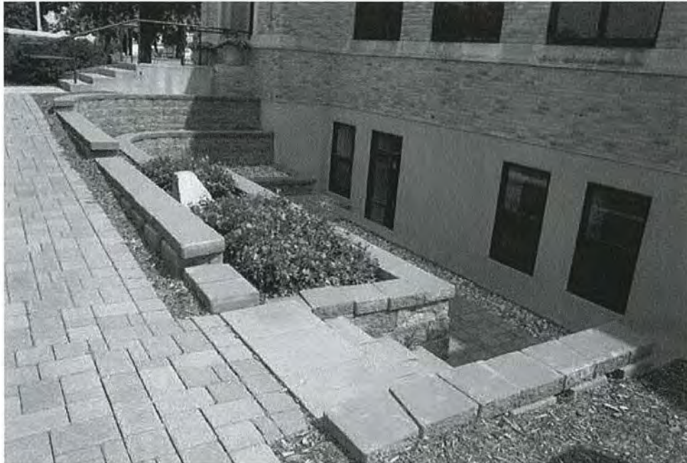
Figure 3: Landscaping on west façade with basement door. Camera facing northeast
