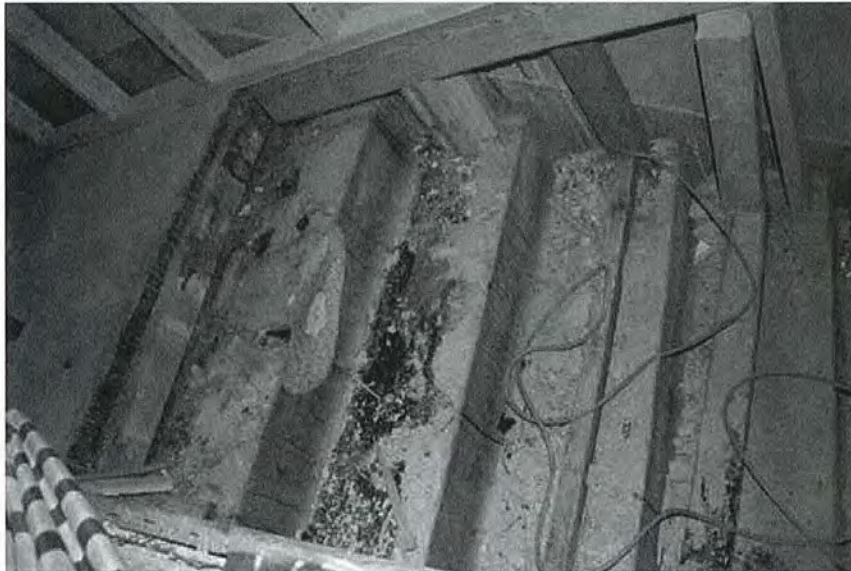
Figure 12: Detail showing stairs inside basement storage room.
