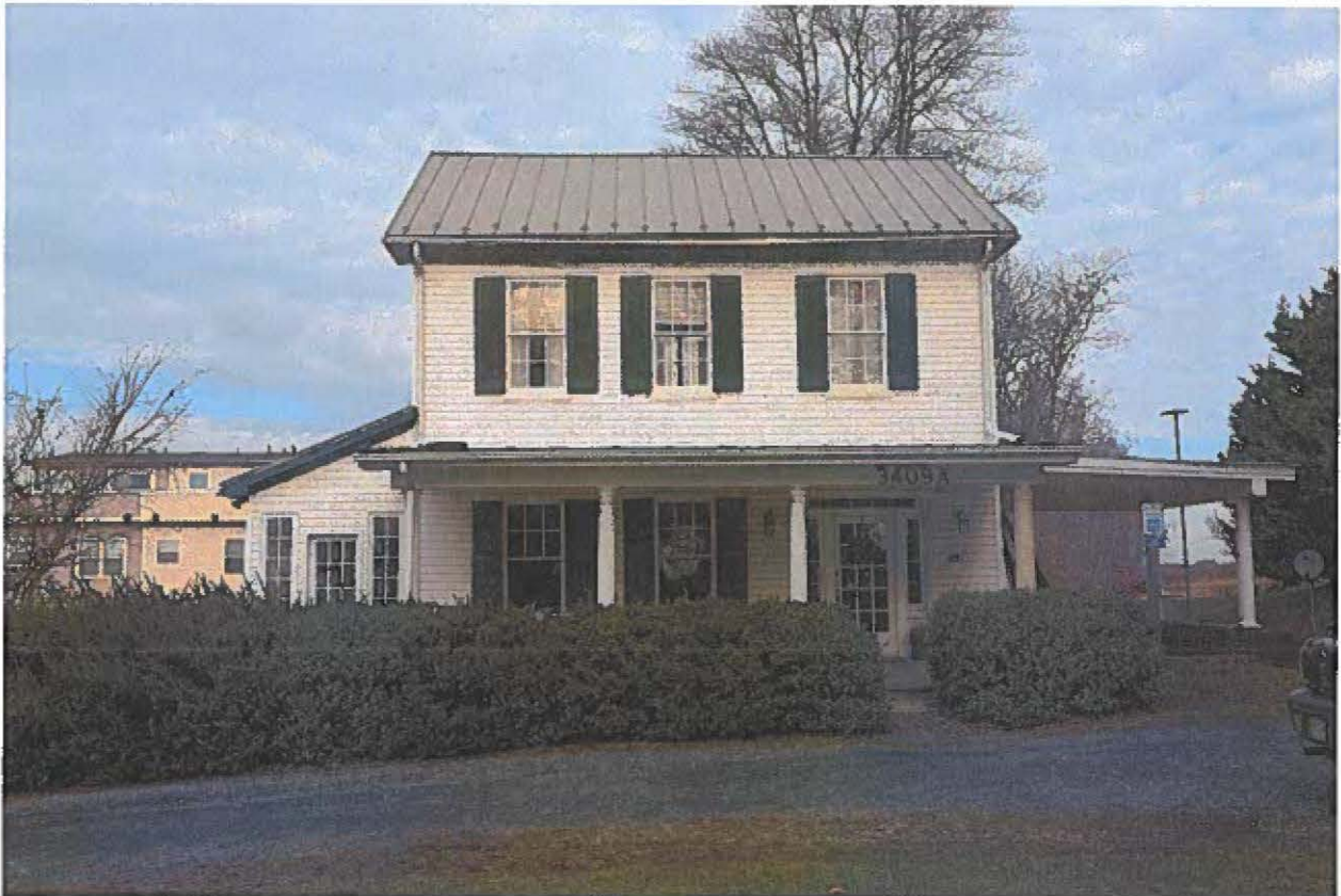
MD_FrederickCounty_Cockey'sHouseandStore_0002.tif Cockey/Jamison/Hendrickson House, south front elevation
