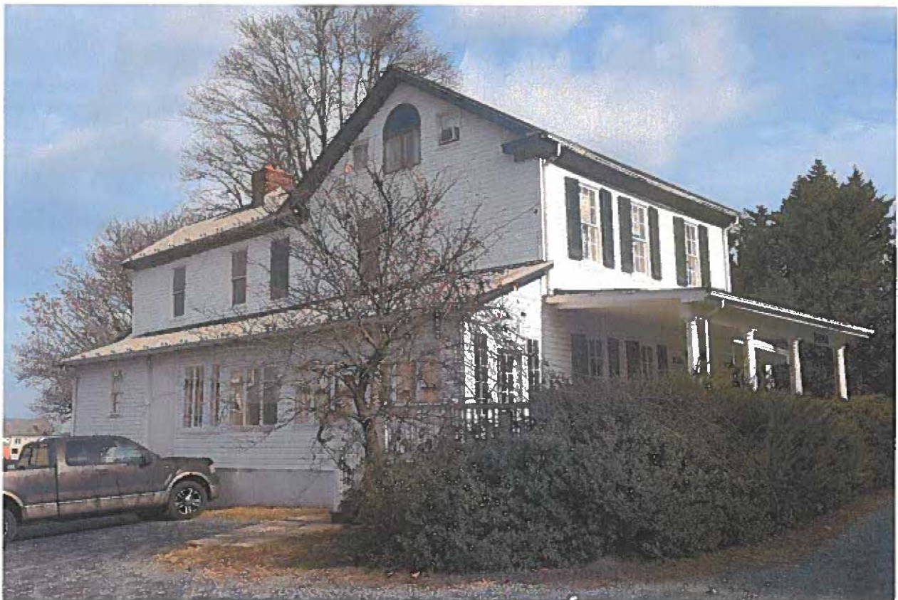
MD_FrederickCounty_Cockey'sHouseandStore_0003.tif Cockey/Jamison/Hendrickson House, west side elevation
