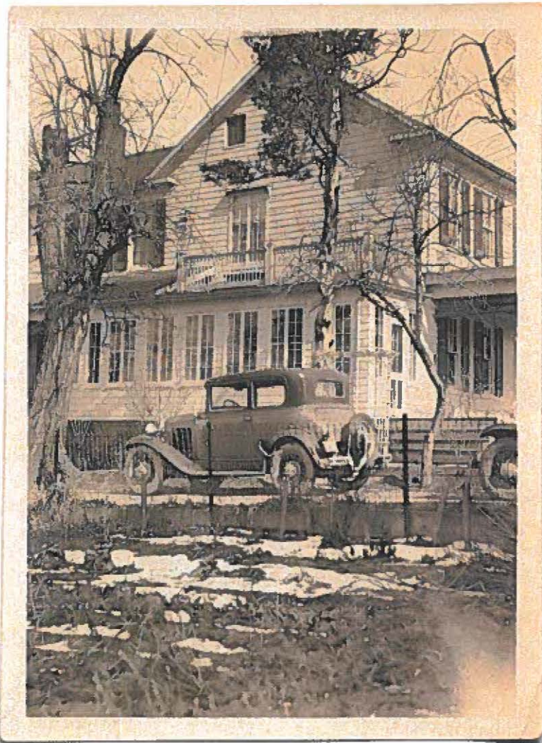
MD_FrederickCounty_Cockey'sHouseandStore_0040.tif Cockey/Jamison/Hendrickson House (Hendrickson home) c.1935, west side, showing new deeper sun porch
