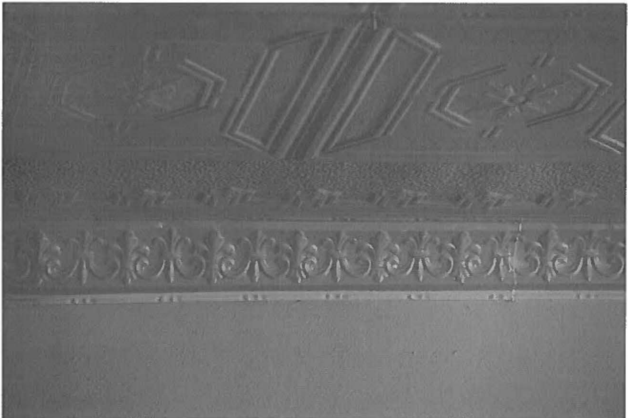
MD_FrederickCounty_Cockey'sHouseandStore_0034.tif Store interior, detail of pressed metal ceiling and cornice
