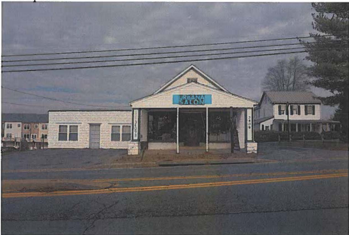
MD_FrederickCounty_Cockey'sHouseandStore_0001.tif Cockey/Jamison/Hendrickson House (right) and Store (left) south facades, from across Urbana Pike
