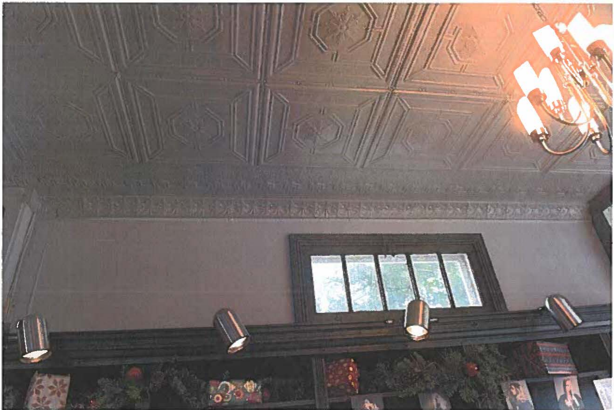
MD_FrederickCounty_Cockey'sHouseandStore_0033.tif Store interior, original pressed metal ceiling
