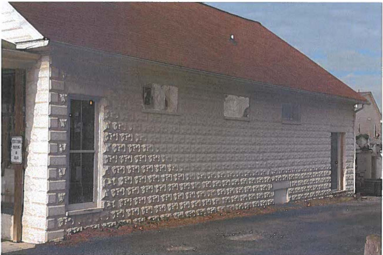
MD_FrederickCounty_Cockey'sHouseandStore_0010.tif Store, east (side) elevation, showing rusticated concrete block construction
