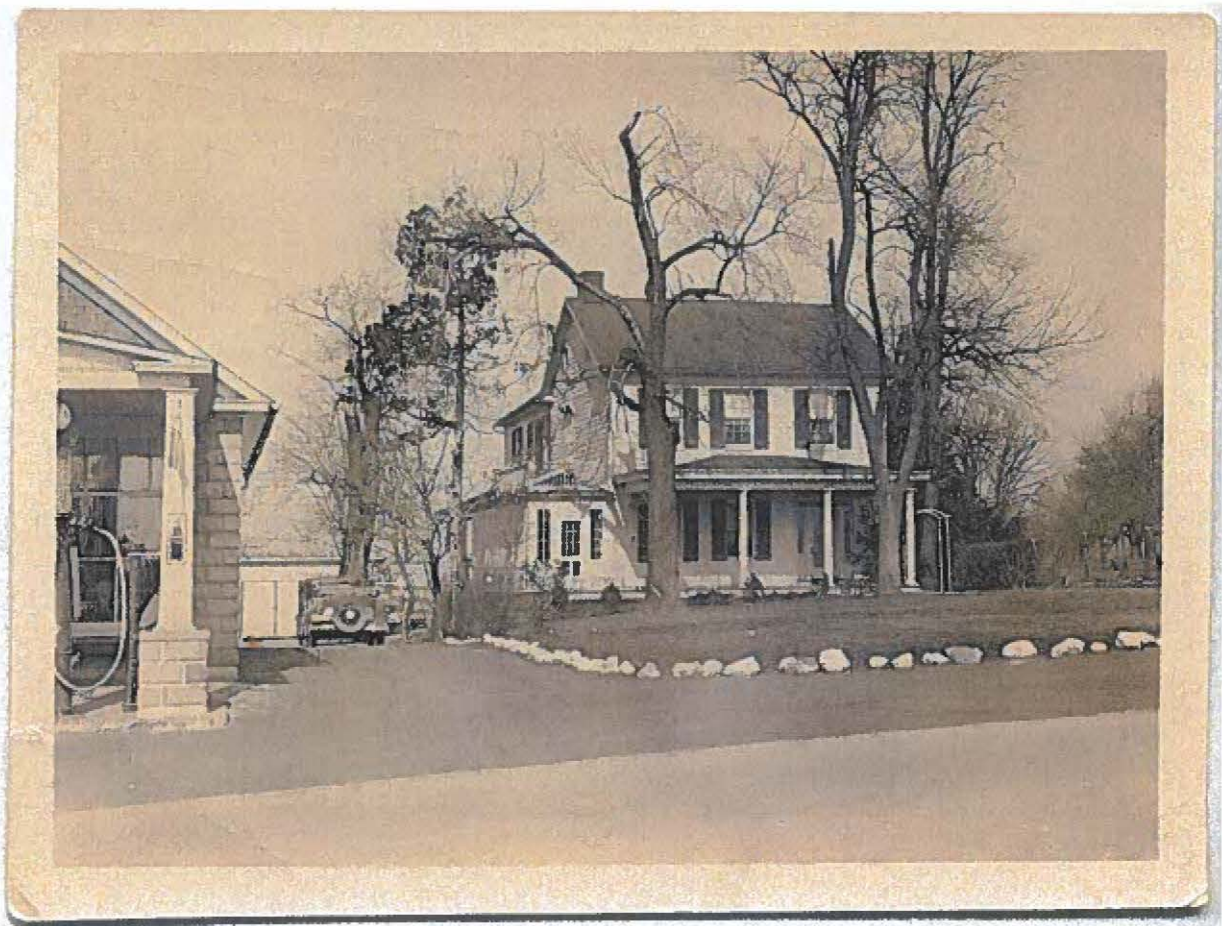
MD_FrederickCounty_Cockey'sHouseandStore_0047.tif Cockey/Jamison/Hendrickson House and Store (Hendrickson's Store) c.1930's, south frontage on Urbana Pike
