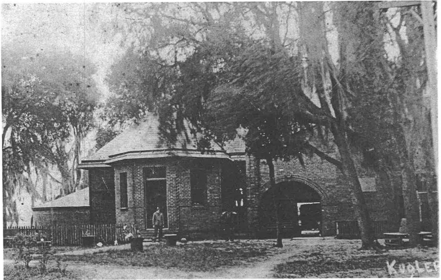
WATERWORKS PARK, PUMPING STATION EARLY TWENTIETH CENTURY/FIGURE 13
