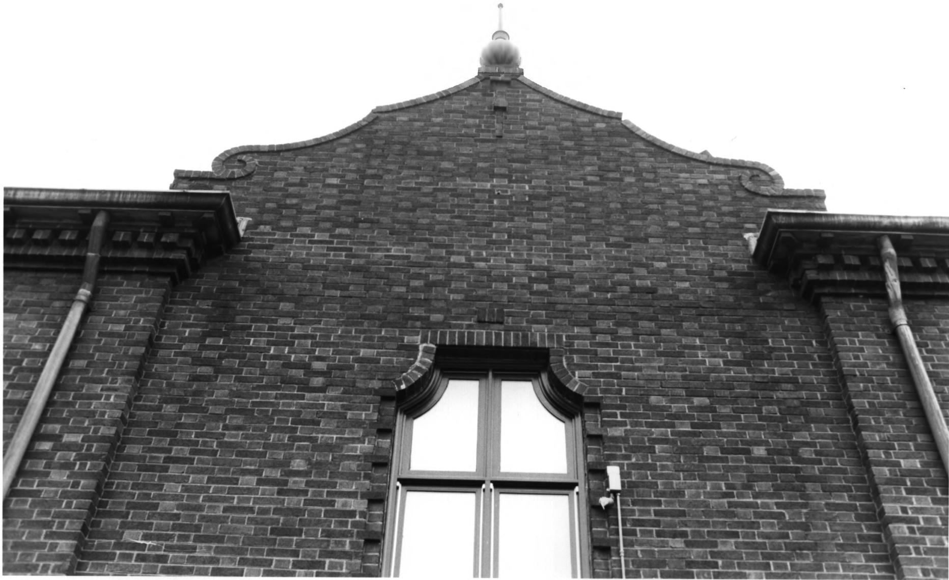
Bovey VILLAGE HALL Bovey, ITASCA CO., MN 010827-7
