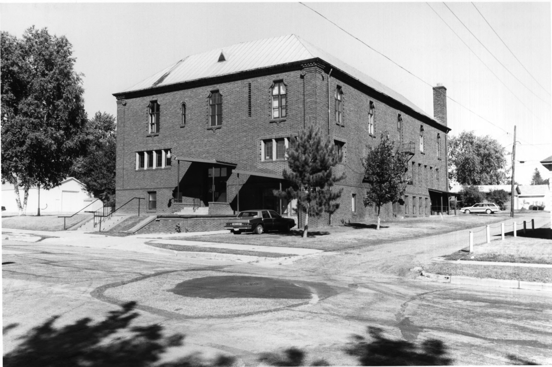
Bovey Village Hall BOVEY, ITASCA CO., MN 010 827-16
