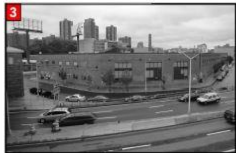
View of the bus depot from the walkway on the Willis Avenue Bridge (Photo, Henry Ballard Terepka).
