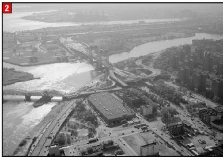
Aerial view of the bus depot looking East towards Randall's Island (Library of Congress).
