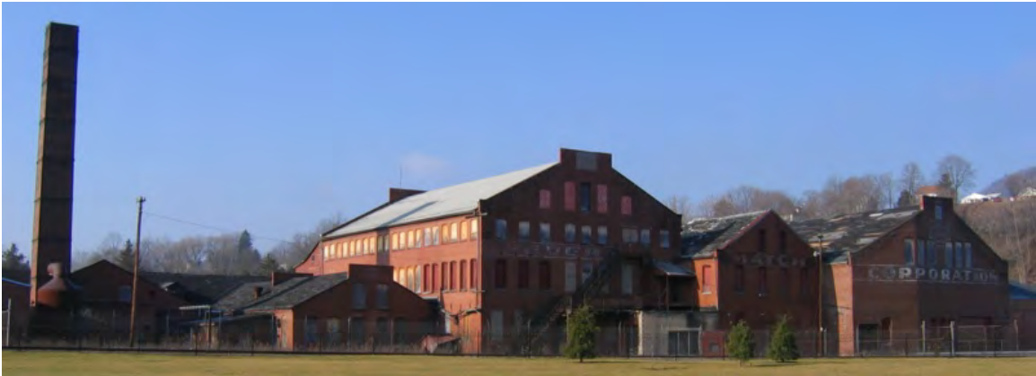
Pennsylvania Match Factory, Bellefonte, PA Constructed 1900, current photograph, shown after clerestory removal Supplemental Photograph #3
