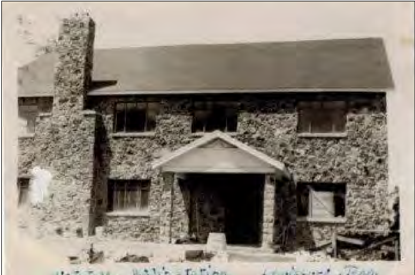
Figure 4. View of WJJM under construction (1946).
