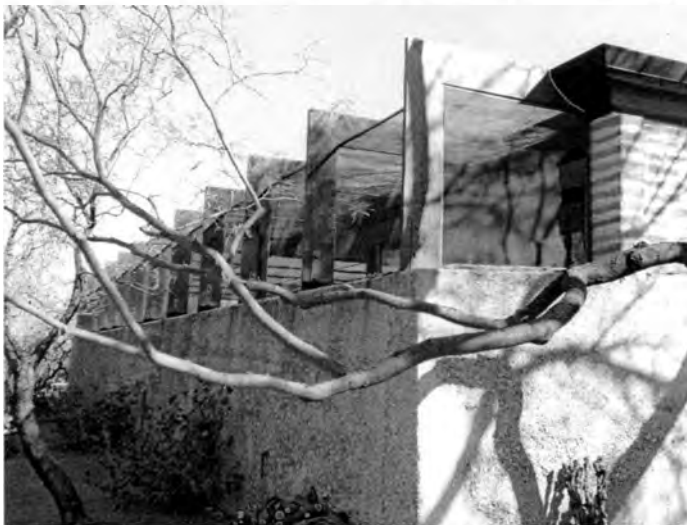
Figure 1: Gist Residence from northeast
