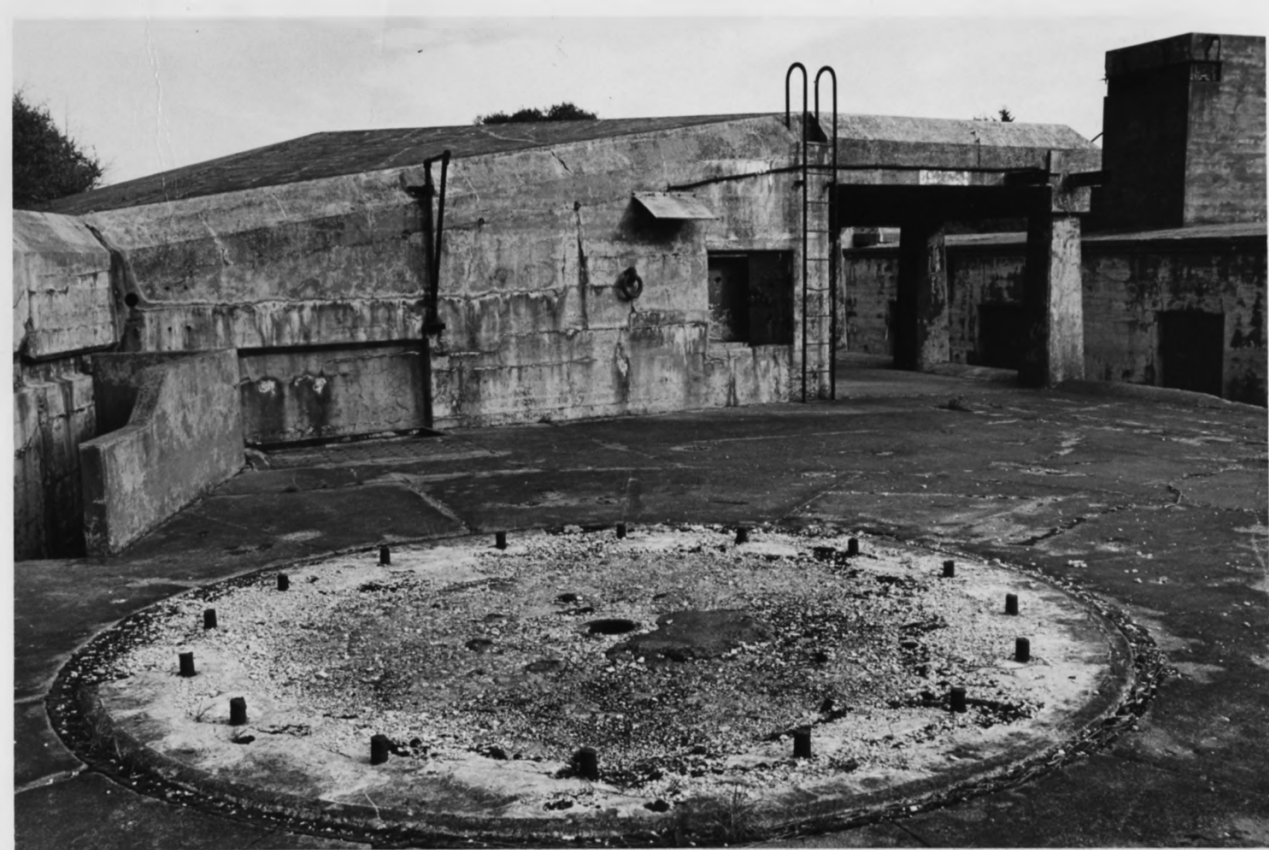
Fort Worden, Armament Emplacement, Port Townsend, Washington October 1975
