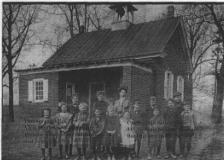
Historic Photograph 9 of 10: This 1904 picture matches the olive photograph in detail and composition. The surrounding vegetation, however, indicates that they were taken at different times of the year. The cornice returns on the east elevation feature profiles different than what are currently in place [also visible in Historic Photograph 8].
