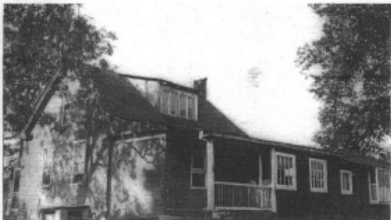
Historic Photograph 10 of 10 This 1938 image of the south and west elevations of the schoolhouse shows a large addition to the south and east. Note the added dormer, rising cupola, and one-over-one window in the south elevation of the extension. There appears to be a rudimentary covering for a bulkhead at the south end of the west elevation.
