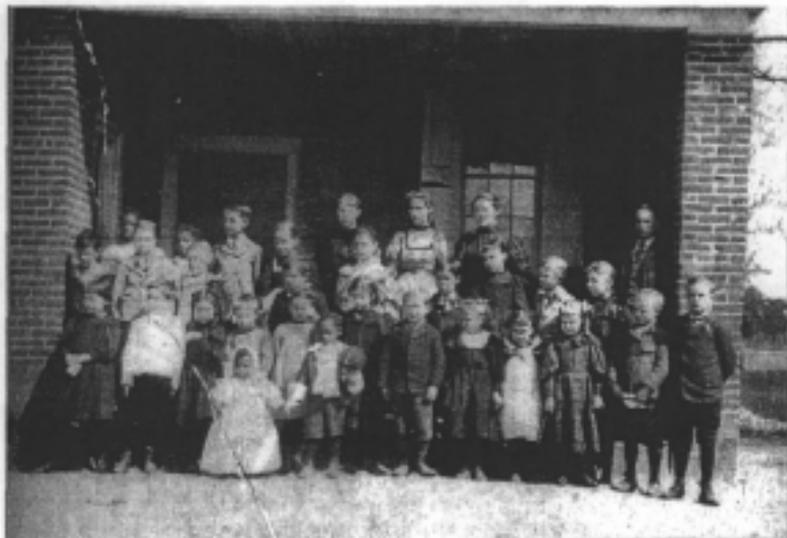
Historic Photograph 3 of 10. To accommodate the children from the first two photographs in a single portrait, this wider image shows the east two bays of the south elevation. Note the width of the primary entry door and the full view of the window and shutters. The framing of the porch roof matches the current configuration.
