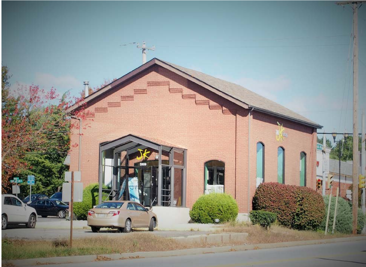
Figure 14, Photo of Lehigh Valley Transit Company Substation, East Norriton, constructed c.1912
