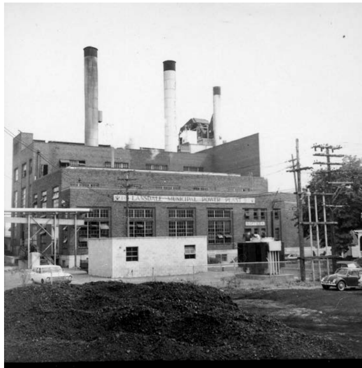
Figure 16, Photo of Lansdale Electric Generating Plant, building in upper photo constructed c.1898. Replaced by building in lower photo, constructed c.1920
