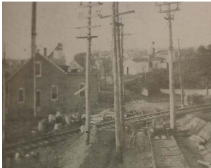
Figure 11, Upper Photo Sellersville Electric Light and Power Generating Plant, constructed c.1900. Lower Photo shows the building on left.
