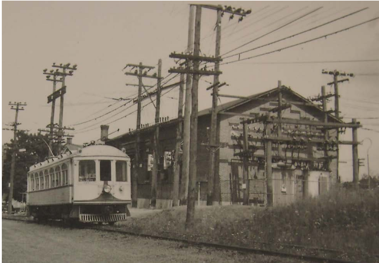
Figure 12, Photo of Sellersville Substation of Lehigh Valley Transit Company, constructed c.1912
