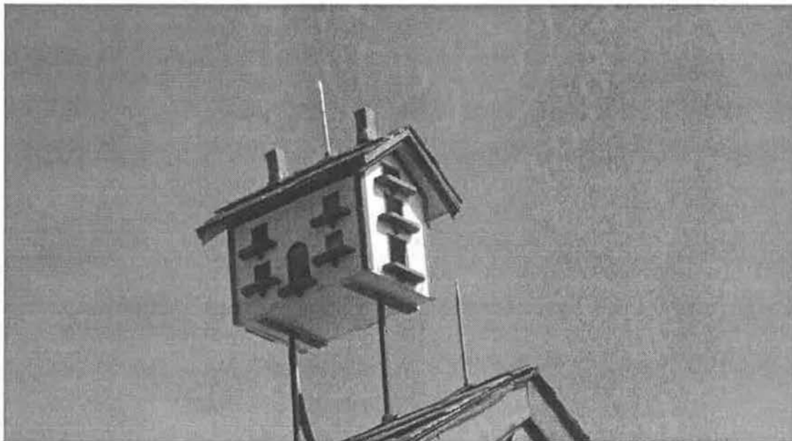
Photo #15 Bird house on Wing. View to northeast, Mar. 2016.
