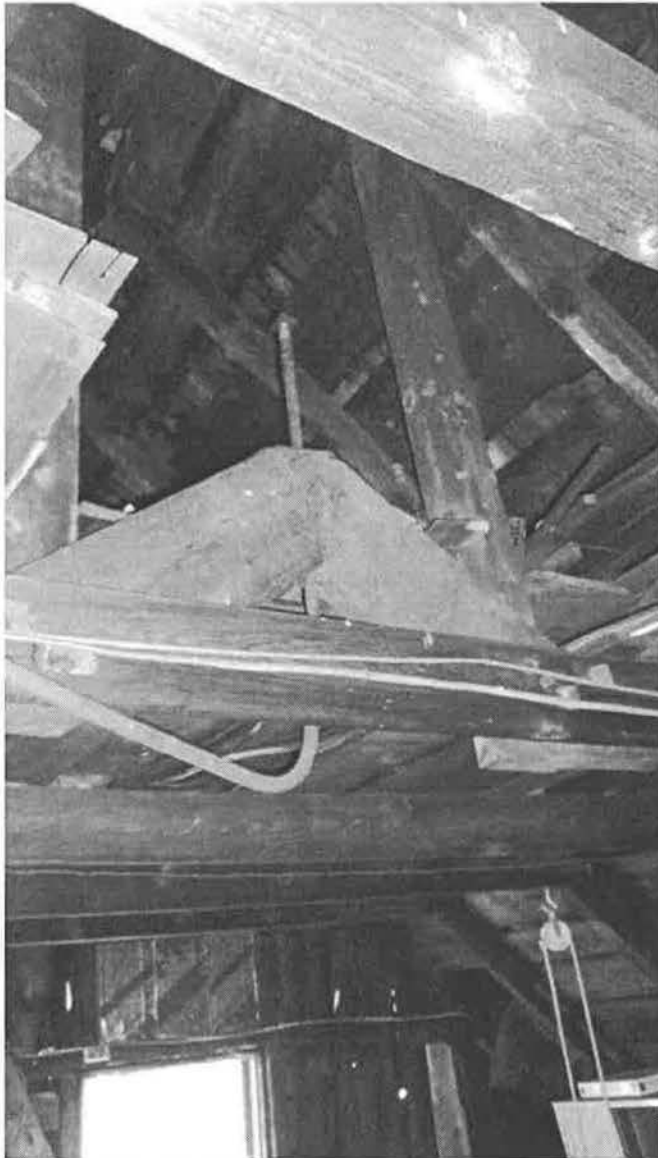
Photo #36 Carriage barn attic – tie-rod and truss. View to east, June 2016.
