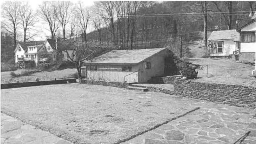
Photo #8, Pool house and lower terrace. View to southeast, Mar. 2016.
