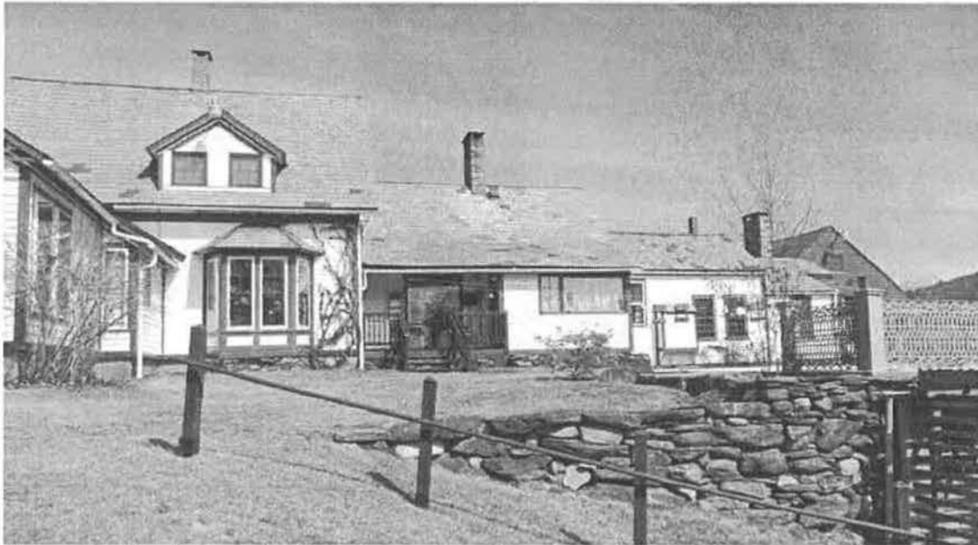
Photo #16 South elevation house and ells. View to north, Mar. 2016.
