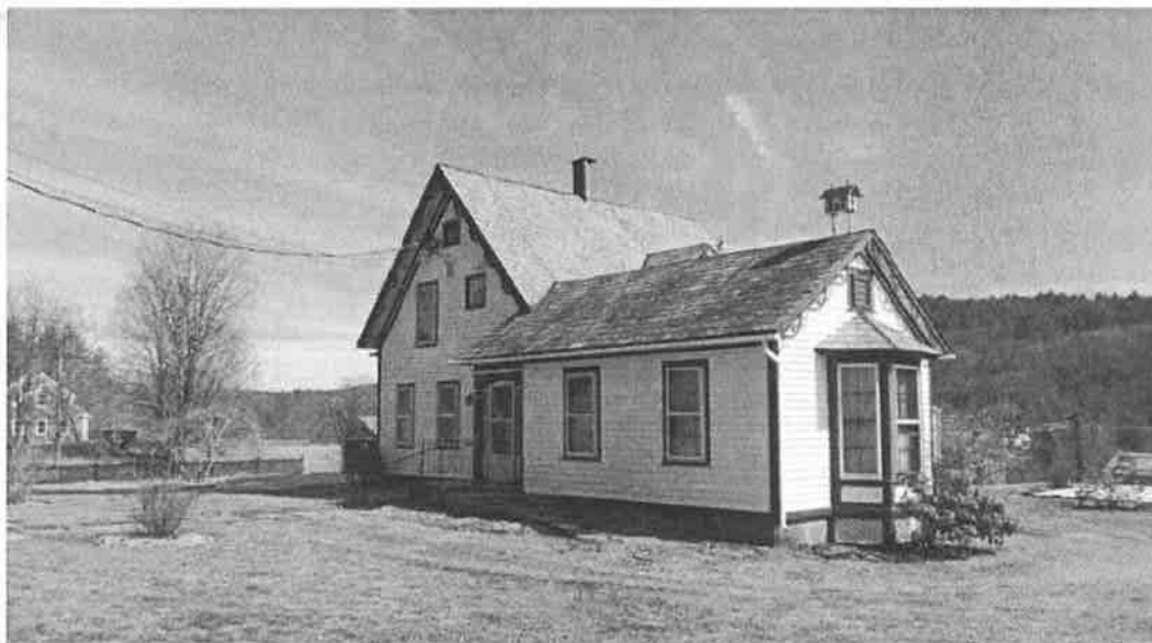
Photo #3. Wing. View to northeast, Mar. 2016.
