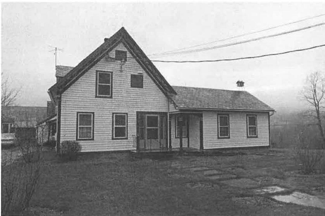
Photo #12 West façade. View to east, Dec. 2015.
