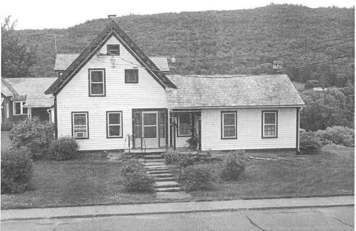
Photo #2. Façade. View to east, July 2016.
