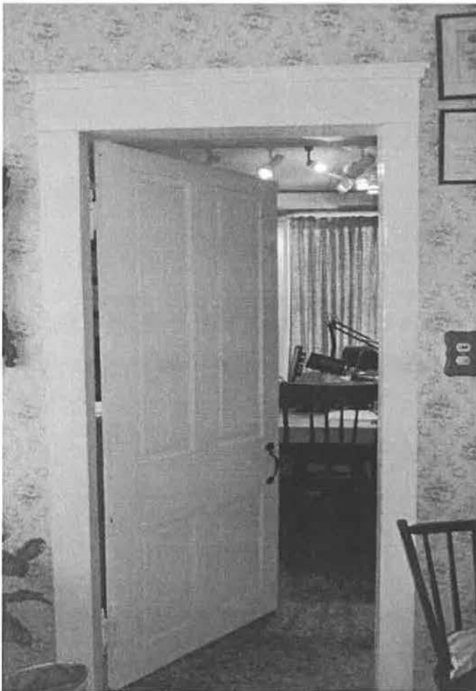
Photo # 20 Door into computer room. View to north, June 2016.
