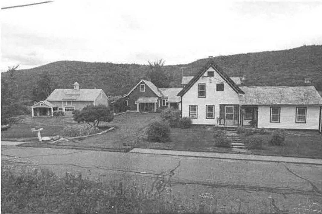
Photo #5. View to east. On left main barn. On right at rear carriage barn and studio, July 2016.
