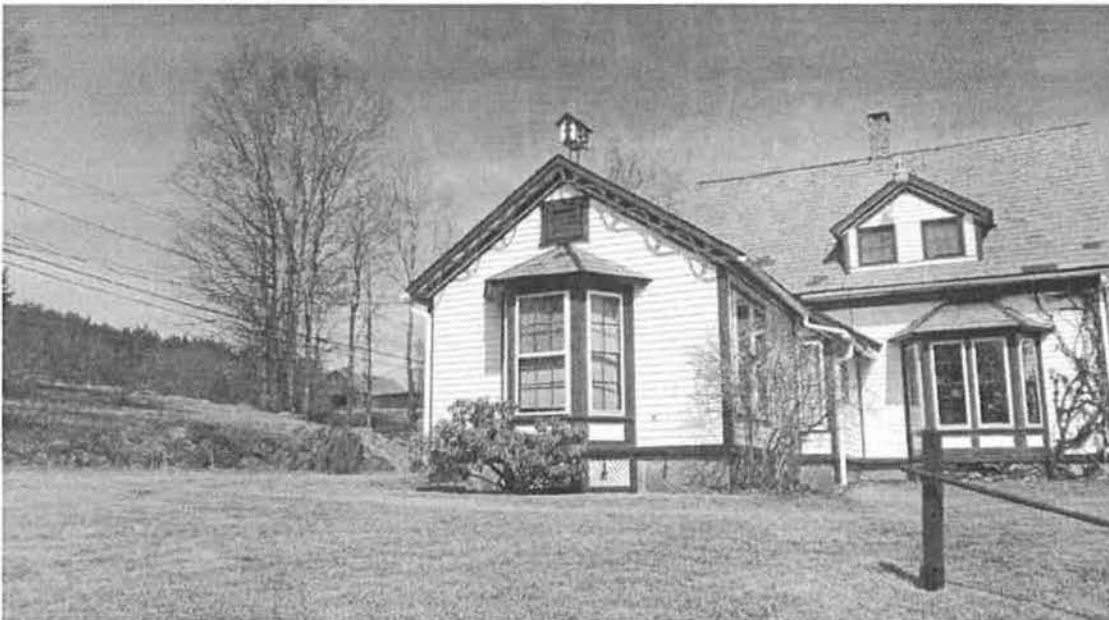
Photo #14 Wing, south elevation. View to north, Mar. 2016.
