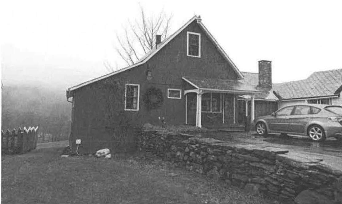
Photo #18 Carriage barn with side aisle and stone embankment. View to east, Dec. 2015.
