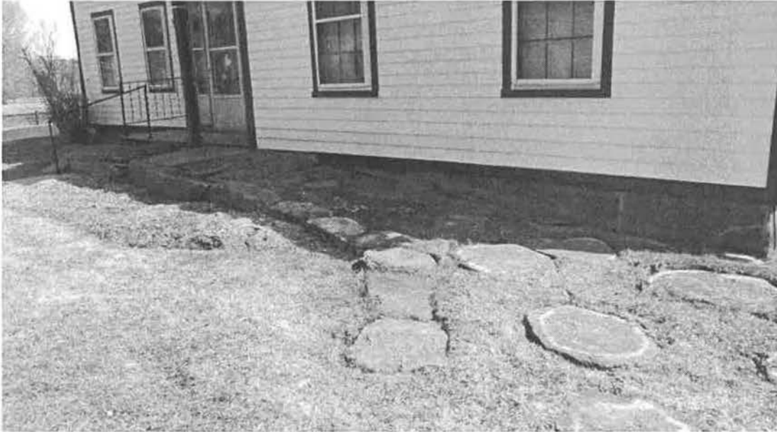
Photo #13 Stone ramp. View to north, Mar. 2016.
