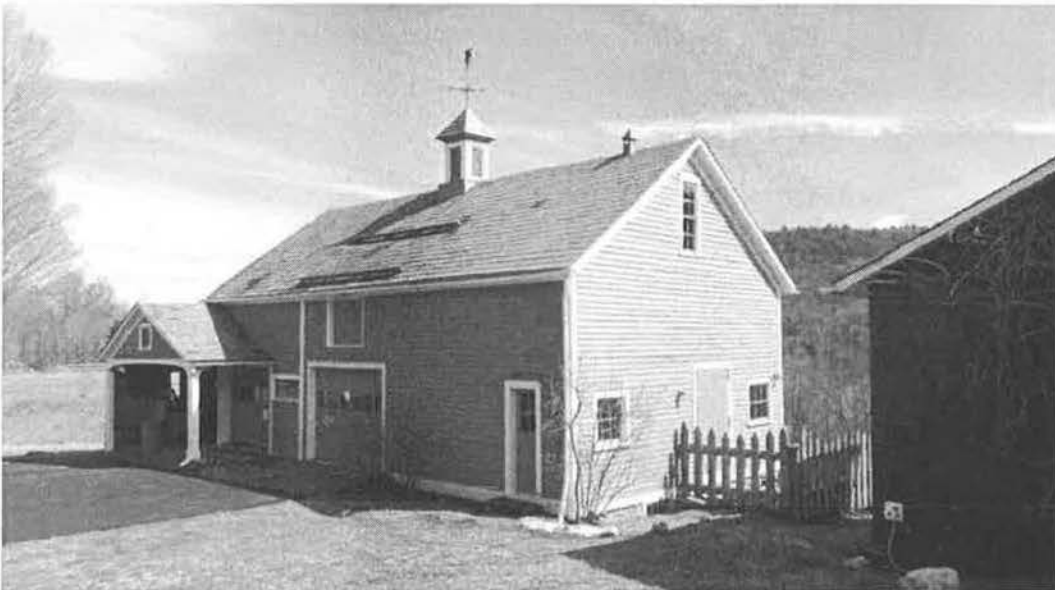
Photo #6. Main barn. View to northeast, Mar. 2016.
