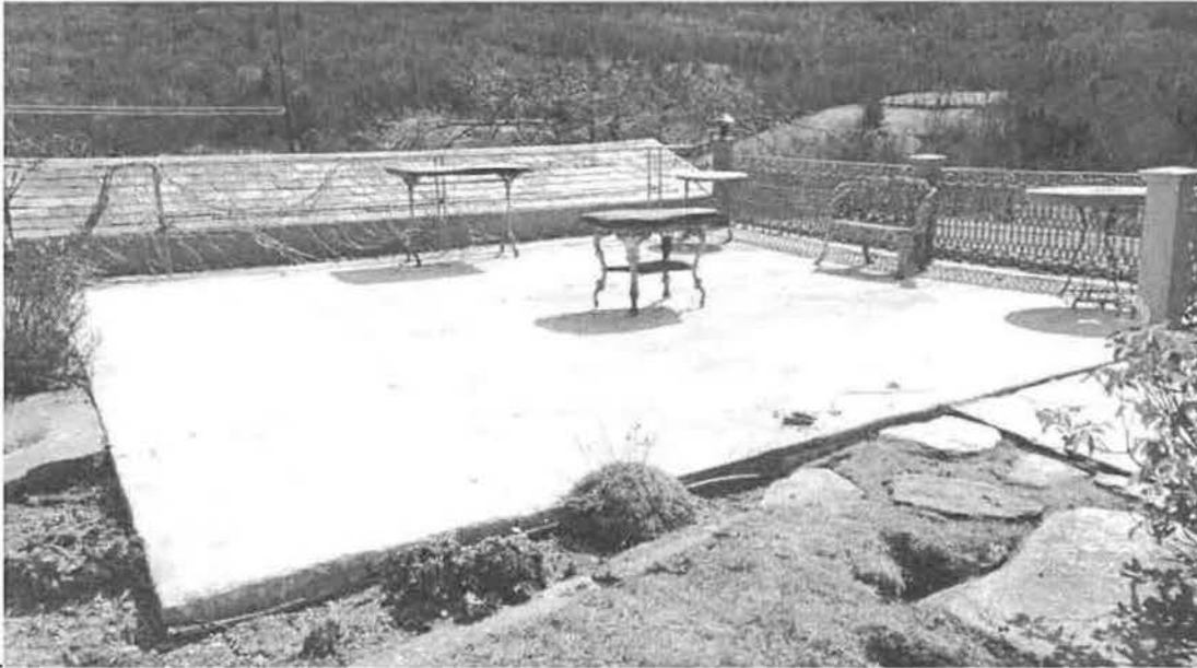
Photo #9. Upper terrace. View to southeast, Mar. 2016.
