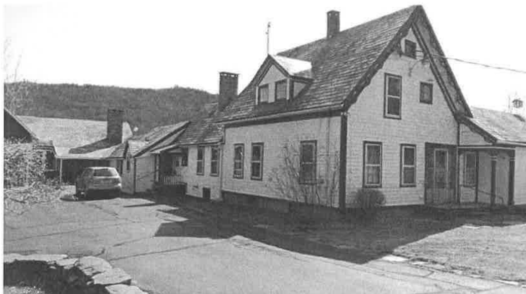
Photo #4. View to southeast of house with two ells, attached studio and carriage barn at rear, Mar. 2016.
