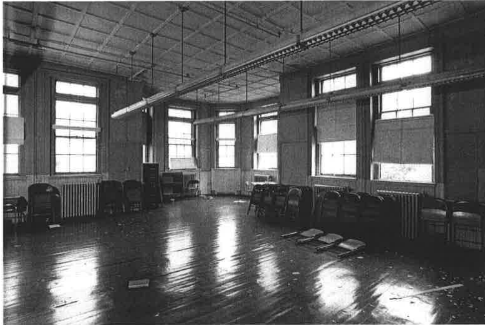
Slater School Classroom, Second Floor, SE Corner with tower Patricia Fisher, Photographer, July 1986
