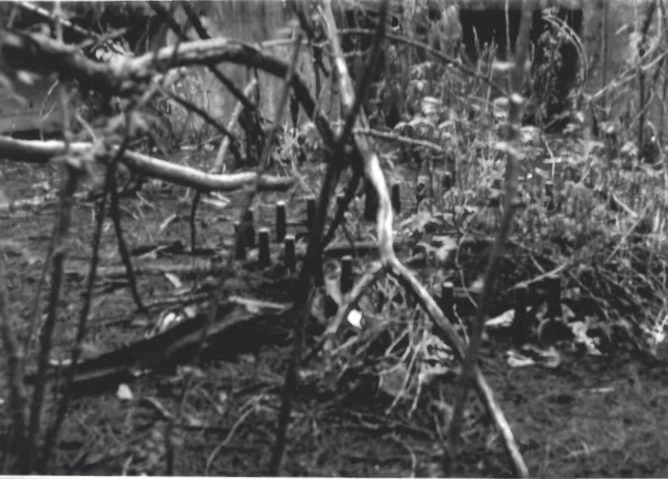
Bolts for the carriage of a 3-inch naval gun, Sand Island, Midway.
