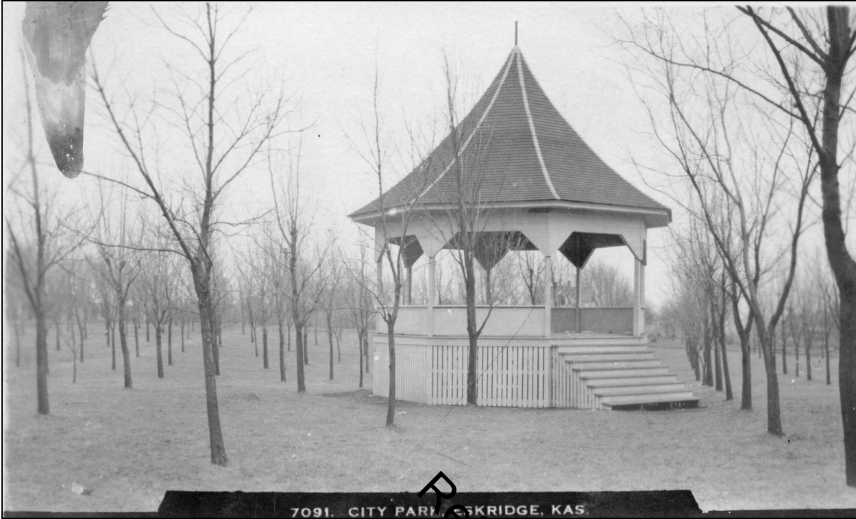
Figure 4. City Park Bandstand, Eskridge, Kansas, c.1908.
