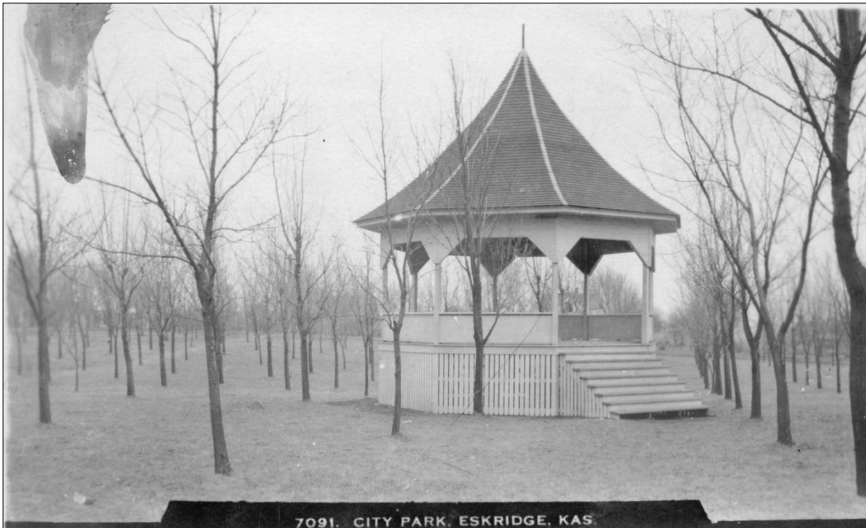
Figure 5. City Park Bandstand, Eskridge, Kansas, c.1908.
