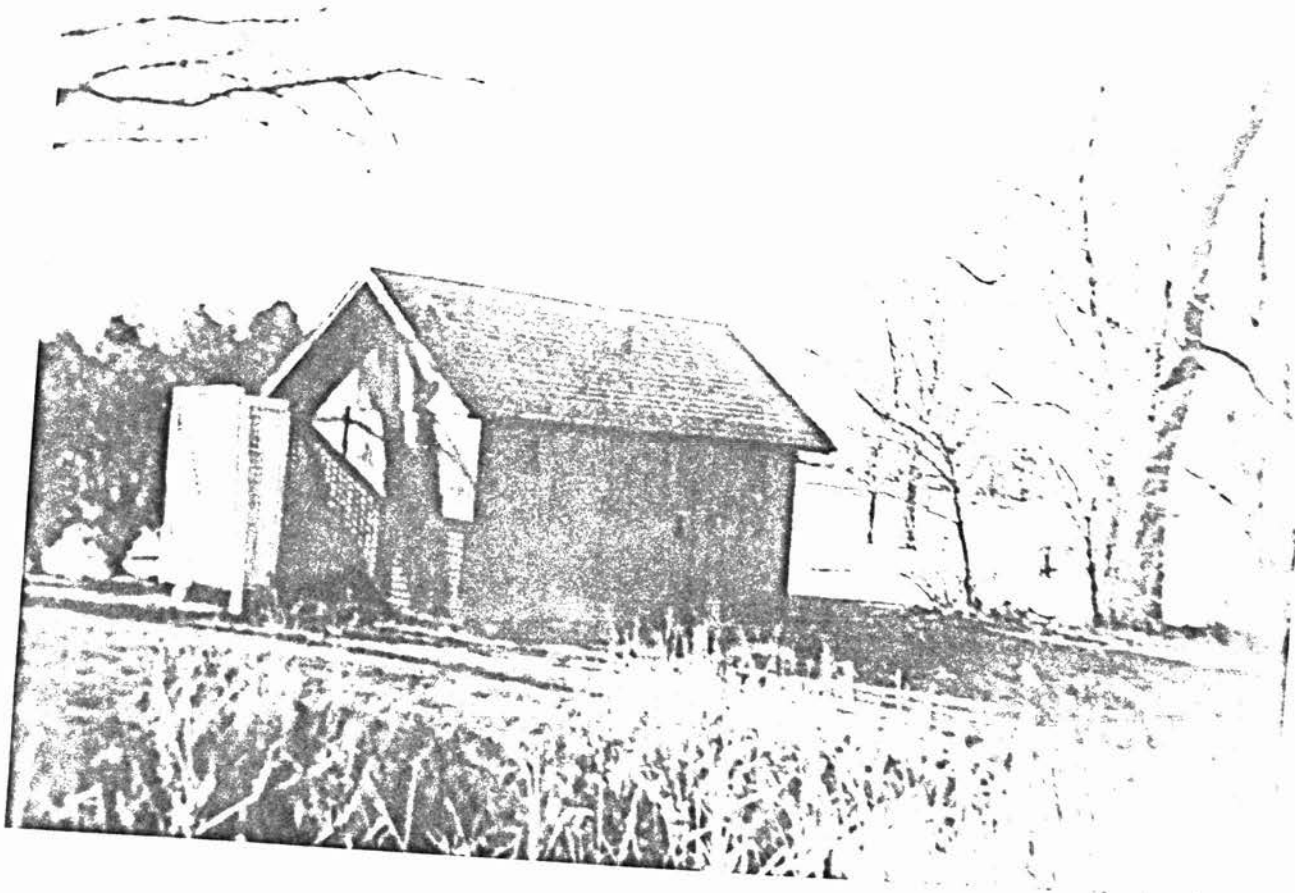
Bldg. No. 55 - Comfort Station Park, General Northeast Elevation Photo: 11/21/74
