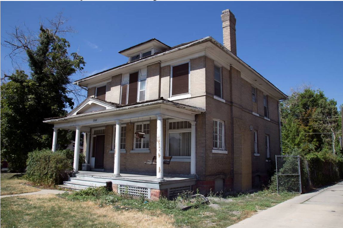
2 of 20. Northeast façade. Camera facing southwest.
