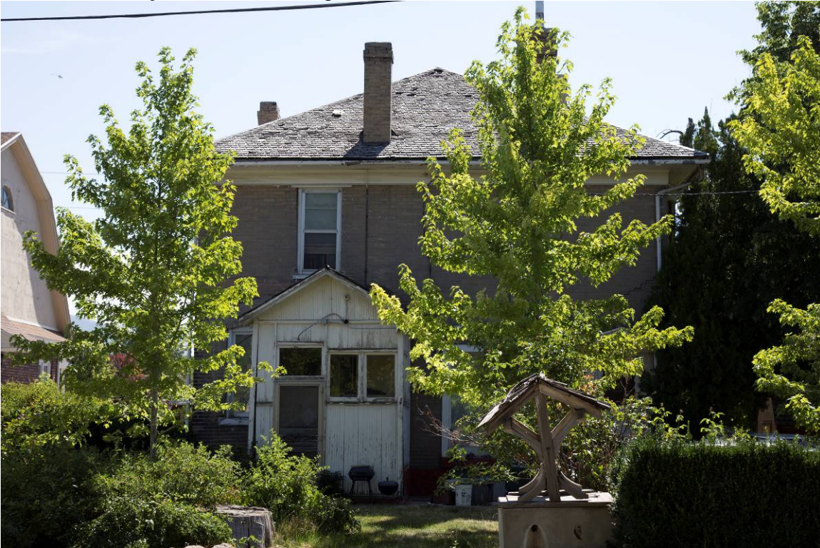
5 of 20. West façade. Camera facing east.
