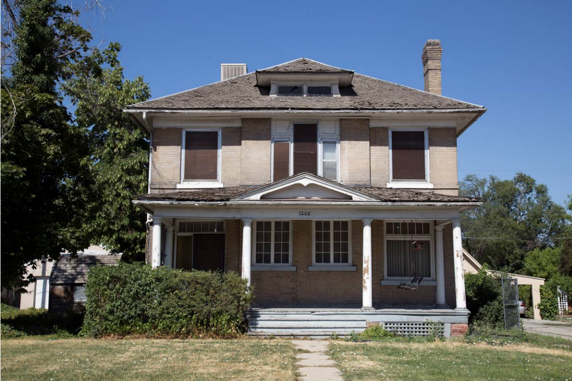
1 of 20. Front (east) façade. Camera facing west.
