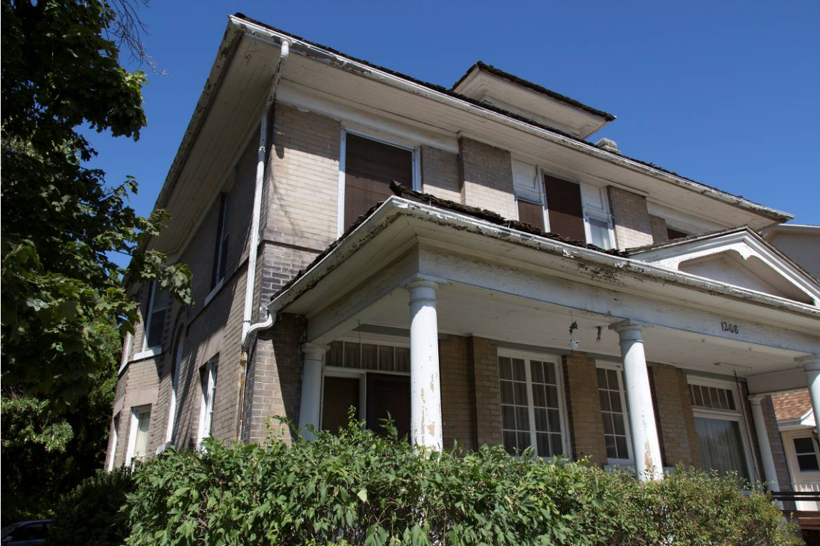
9 of 20. Southeast façade. Camera facing northwest.
