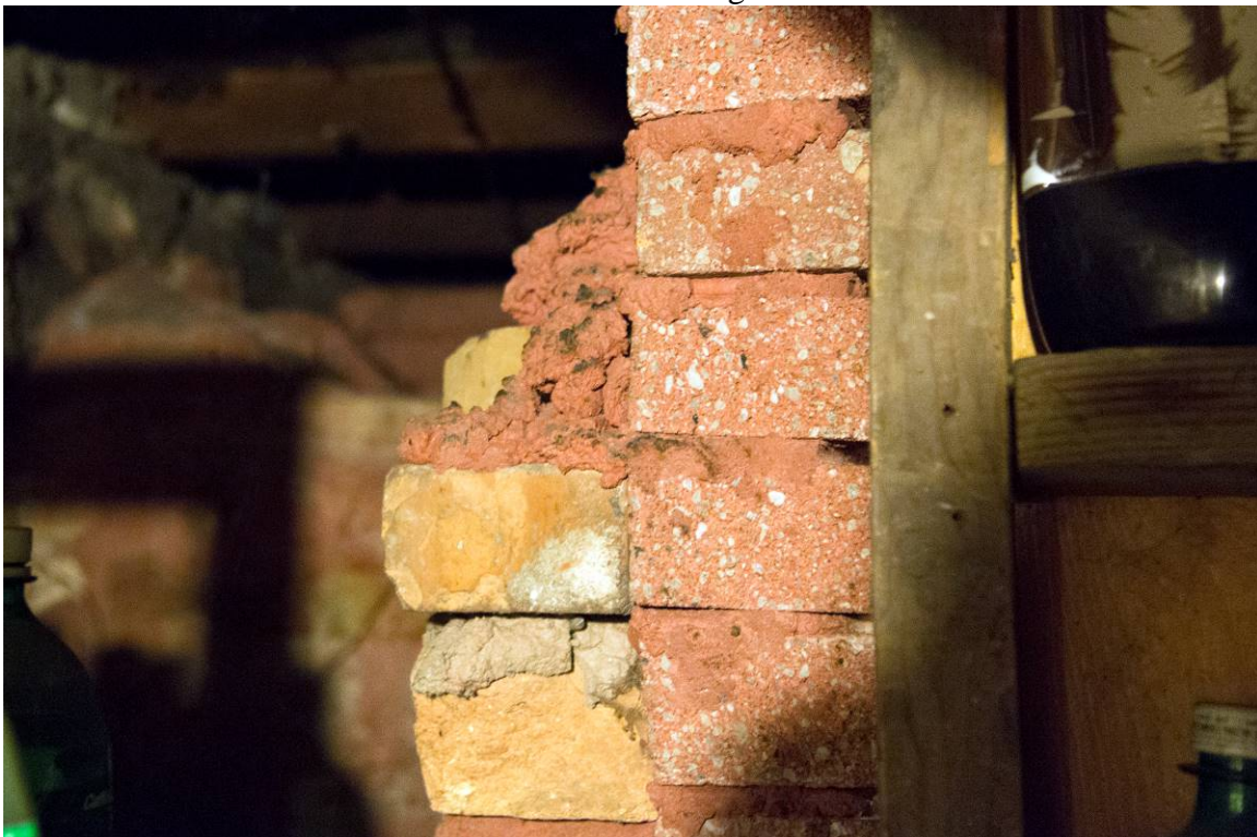
16 of 20. Foundation and brick detail. Camera facing west.
