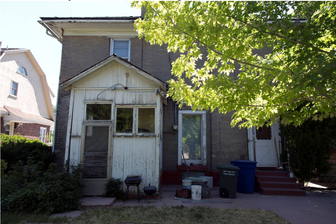
6 of 20. Enclosed porch addition. Camera facing east
