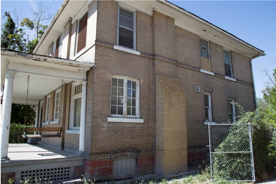
3 of 20. North façade. Camera facing south.
