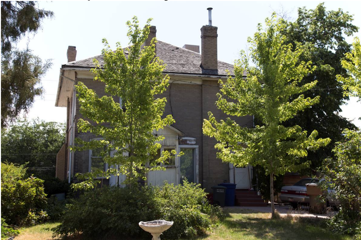
4 of 20. Northwest façade. Camera facing southeast.
