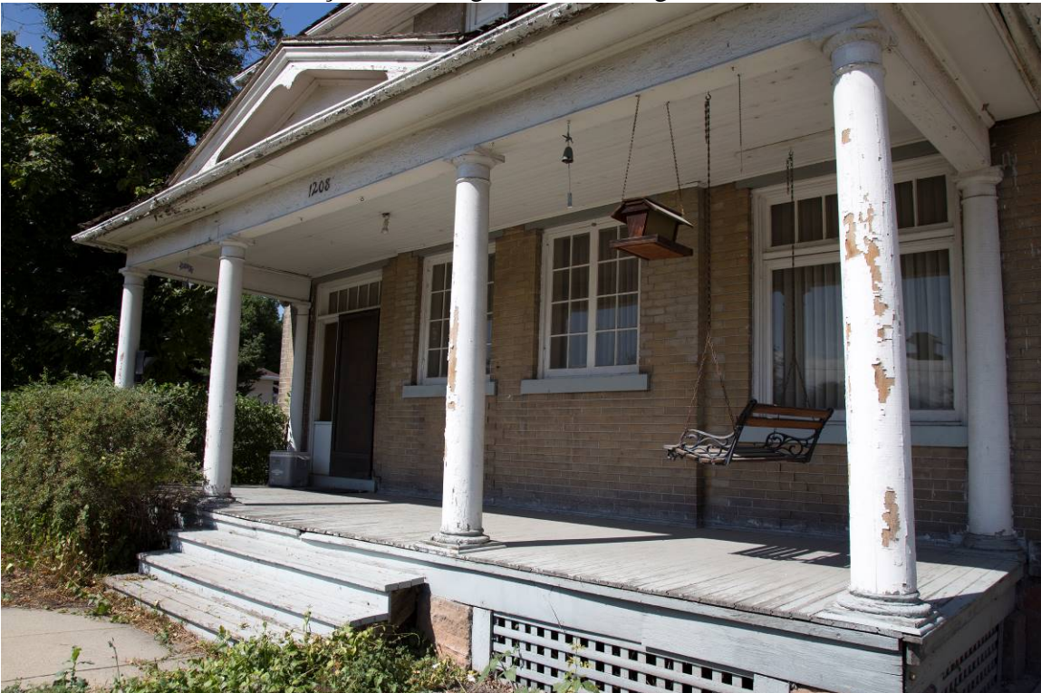
10 of 20. Porch and front façade detailing. Camera facing southwest.
