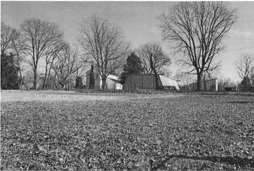
Additional Photo #7. View Toward Main House, Machine Shed, and Chicken Coop, Photographer Facing Northeast.
