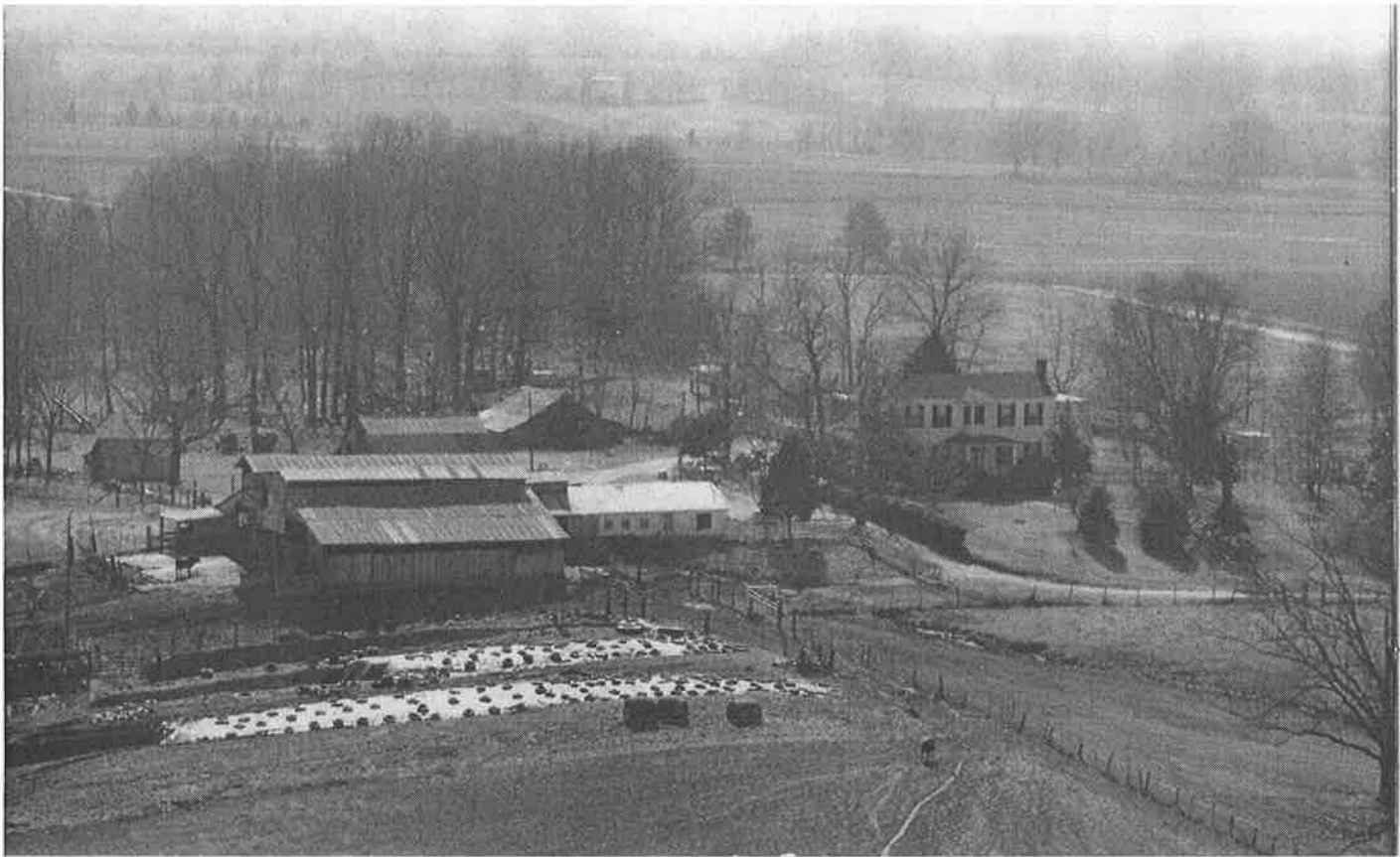
Figure 1. Aerial overview of the farm, c. 1980. Note the silage pits visible in the foreground, north of the barn.
