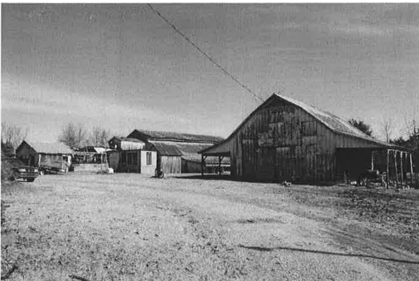
Additional Photo #6. Agricultural Complex (Granary, Barn, Dairy Parlor, Smoke House, and Well House), Photographer Facing Northeast.
