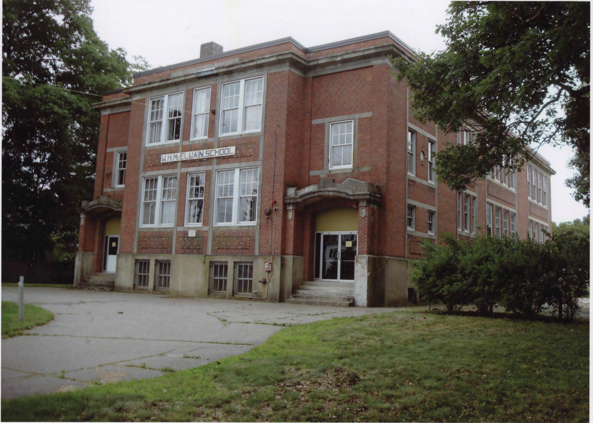
1. North and west elevations (Photographer: Jennifer M. Goldson, 2010)
