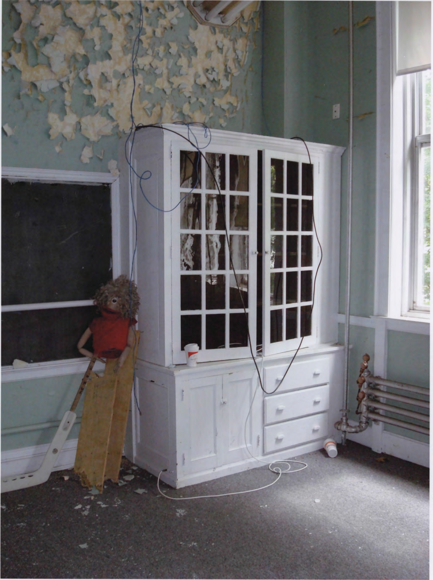
14. Interior - detail of typical cabinet in classroom (Photographer: Jennifer M. Goldson, 2010)
