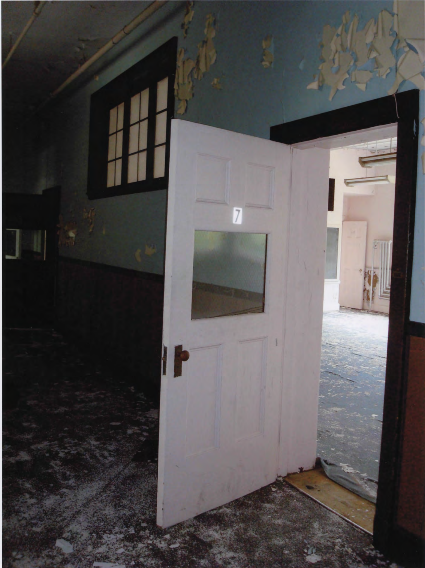
15. Interior - detail of typical classroom door (Photographer: Jennifer M. Goldson, 2010)
