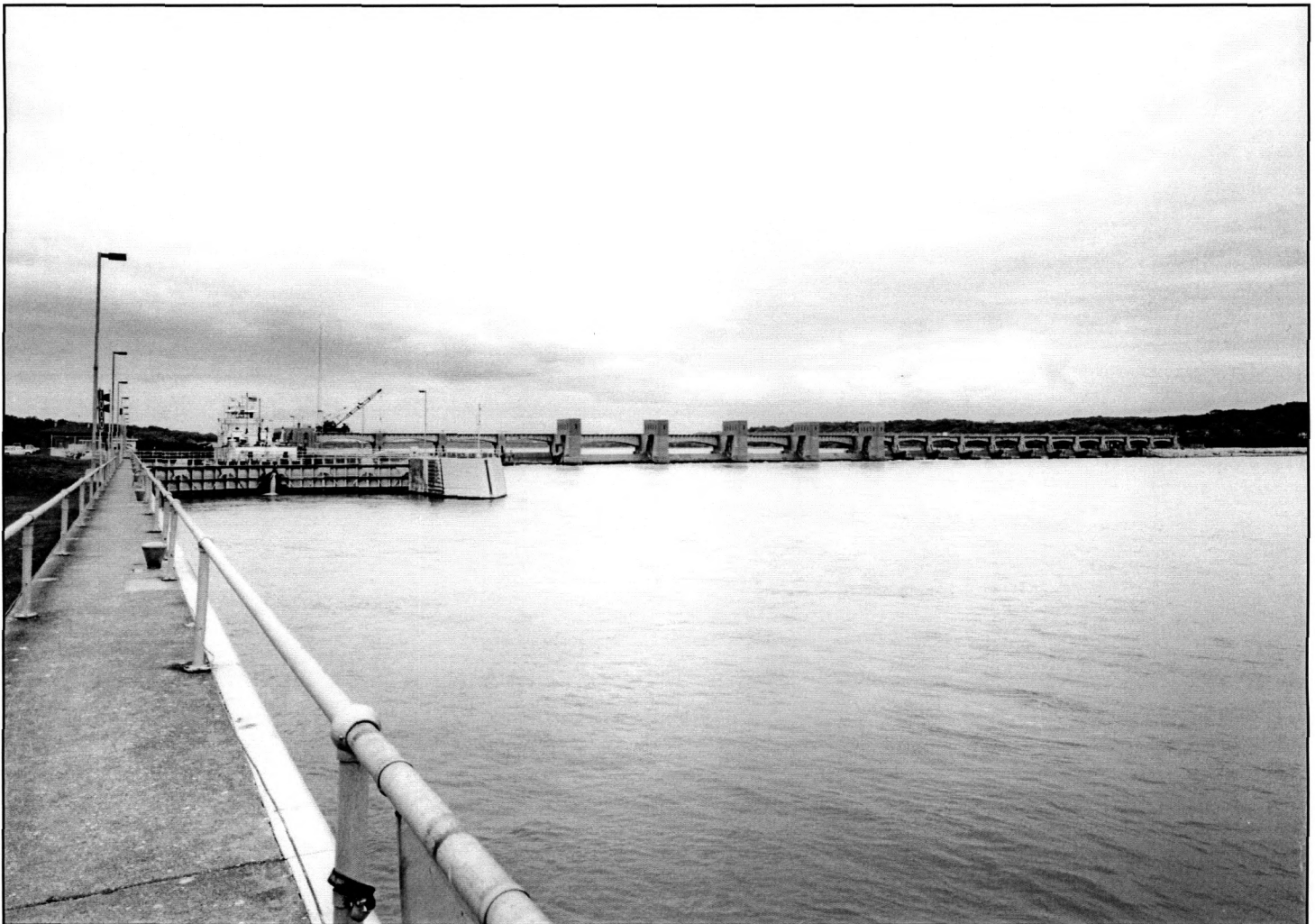
PHOTO 2. General View of Main Lock and Dam, Downstream Side. Photographer: Peter A. Rathbun Date of Photograph: September 1987 Location of Original Negative: IA-25-2, HAER, IOWA, 82-LECLA.V,1- HAER Collection, Prints and Photographs Division, Library of Congress, Washington, D.C. View: From downstream guide wall of the main lock, looking northeast
