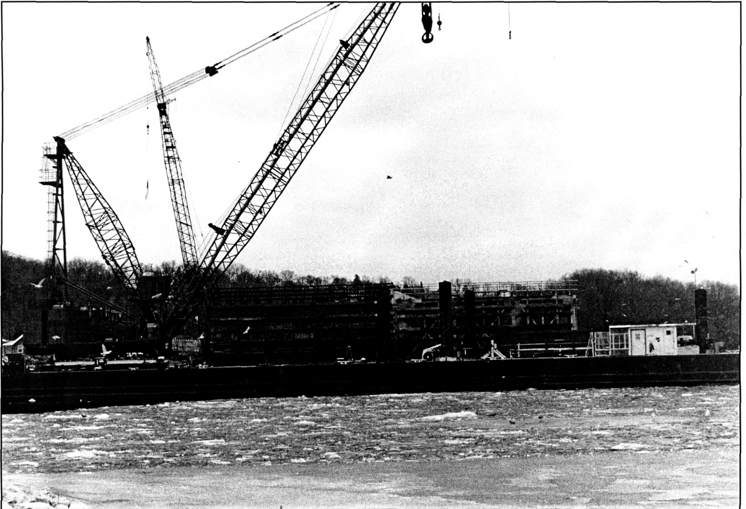
PHOTO 4. One Pair of Main Lock Gates on Work Barge Anchored in the Portion of the Le Claire Lateral Canal Between Smith Island and the Iowa Shore. Photographer: Mary Yeater Rathbun Date of Photograph: February 1998 Location of Original Negative: URM-NATIONAL REGISTER, roll #2, frame 21, Environmental Impact Section, Planning Division, Rock Island District, U.S. Army Corps of Engineers, Rock Island, IL. View: From Le Claire Canal closing dam, looking north
