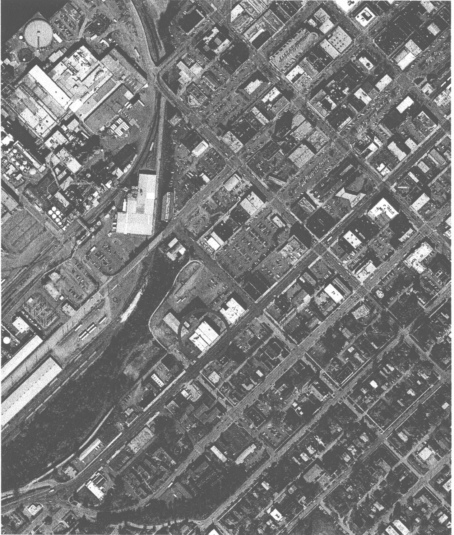
MAP No. 4—SITE VIEW SHOWING THE MORSE HARDWARE COMPANY BUILDING AND SURROUNDINGS.
