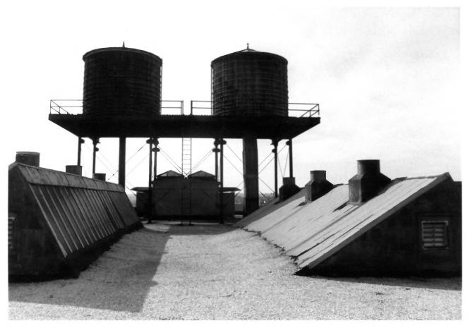
A.K.A. Paca-Pratt Building Dennis P. Dolan Negatives with 110 S. Paca Street Baltimore, Maryland Dennis P. Dolan 23. View looking West across roof of building showing sprinkler system water tanks and roof top sky lights front back and side detail.
