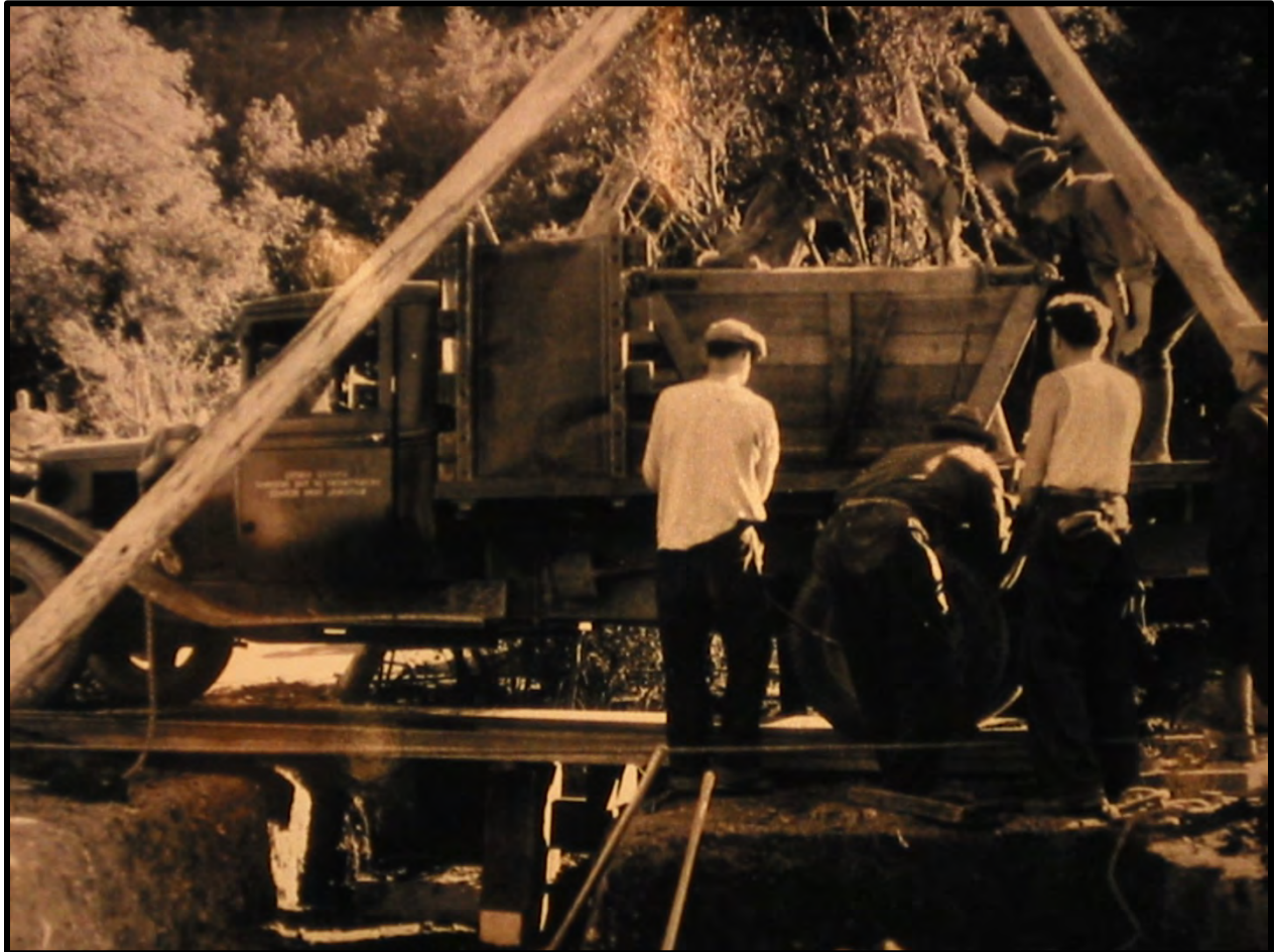
Figure 1. Construction circa 1935. Photo courtesy Mountain Play
