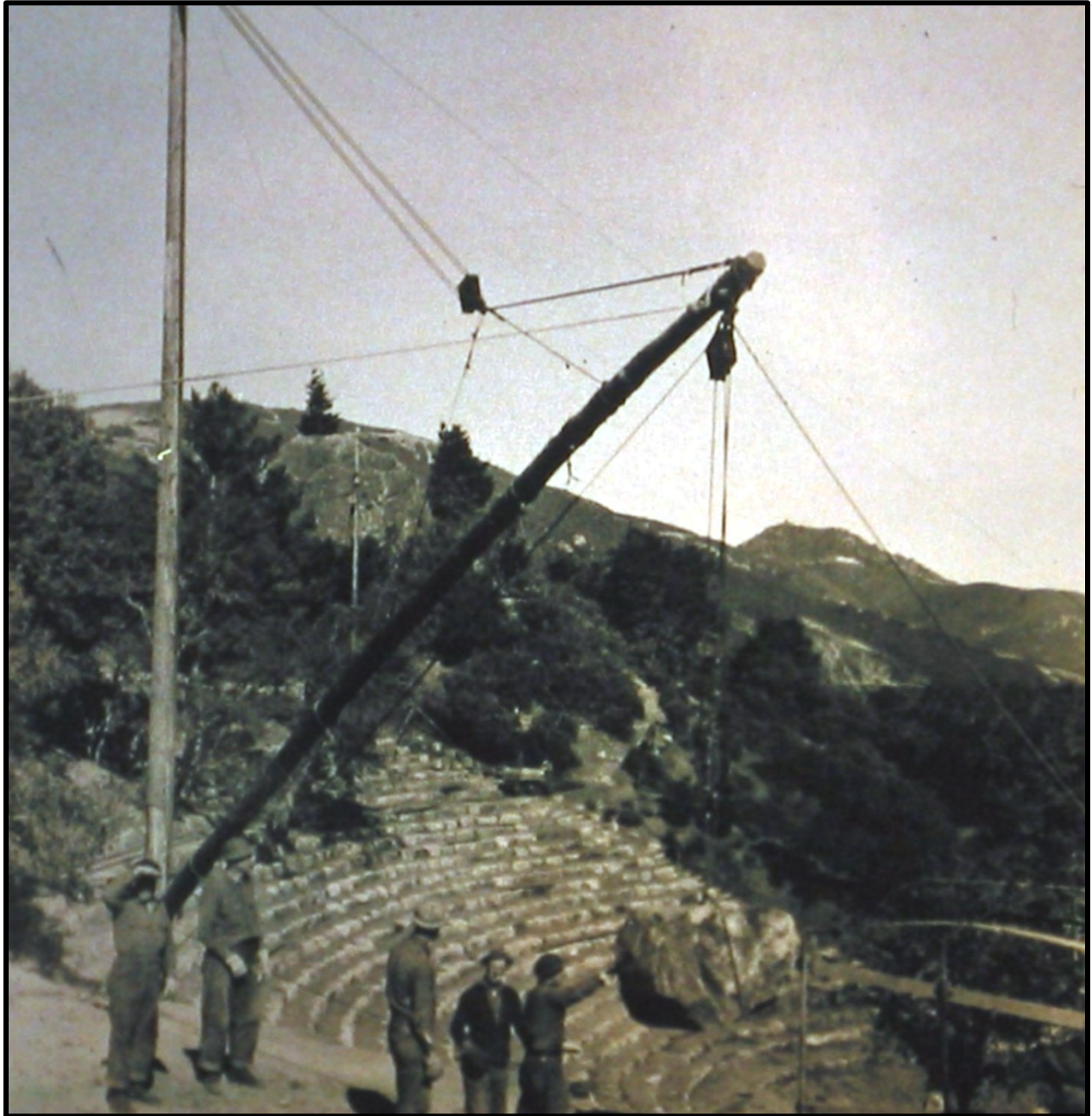
Figure 3. Construction circa 1935. Photo courtesy Mountain Play
