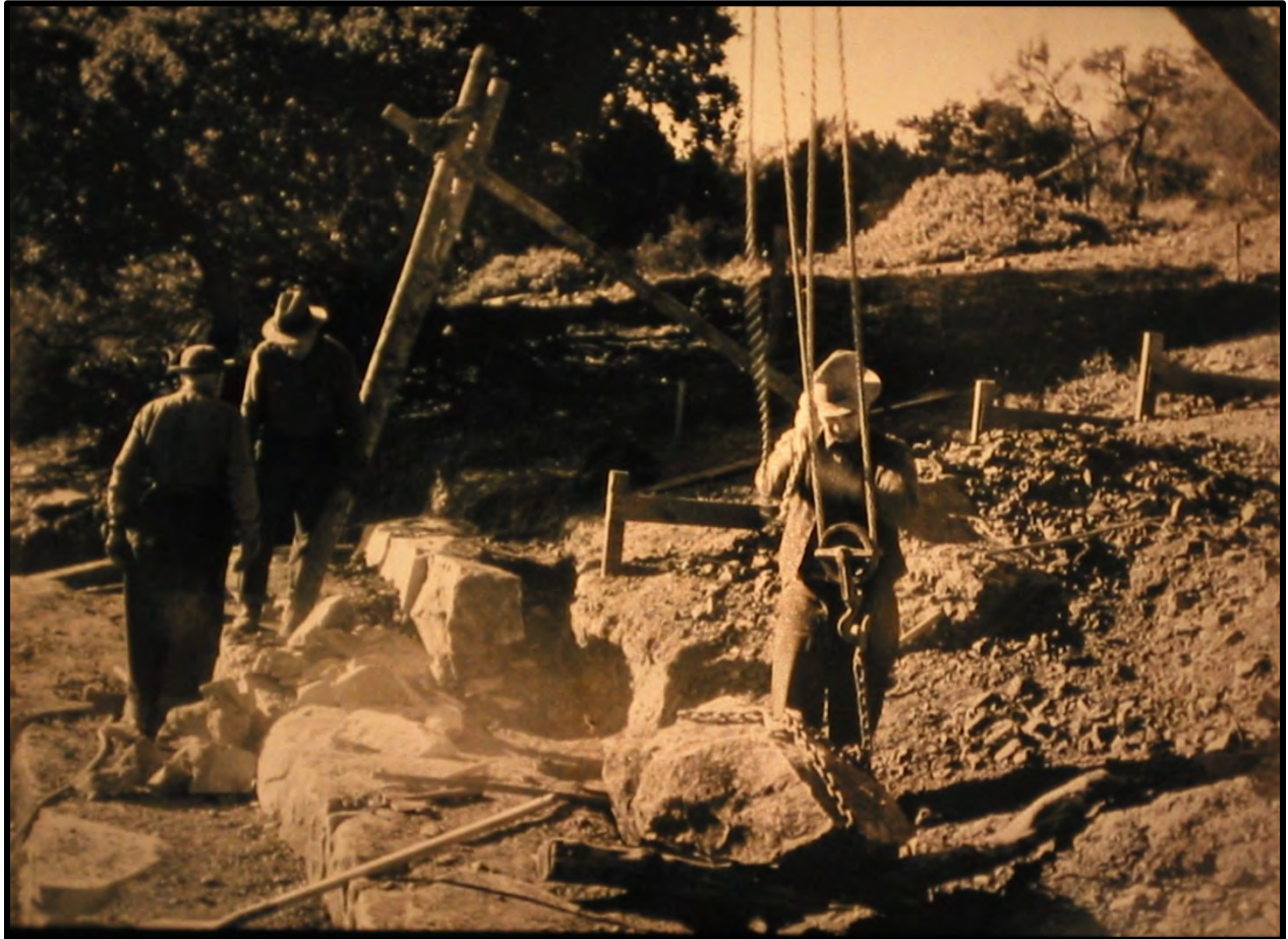
Figure 2. Construction circa 1935. Photo courtesy Mountain Play
